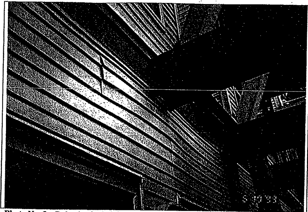
Photo No. 3 – Bulge in vinyl siding.
