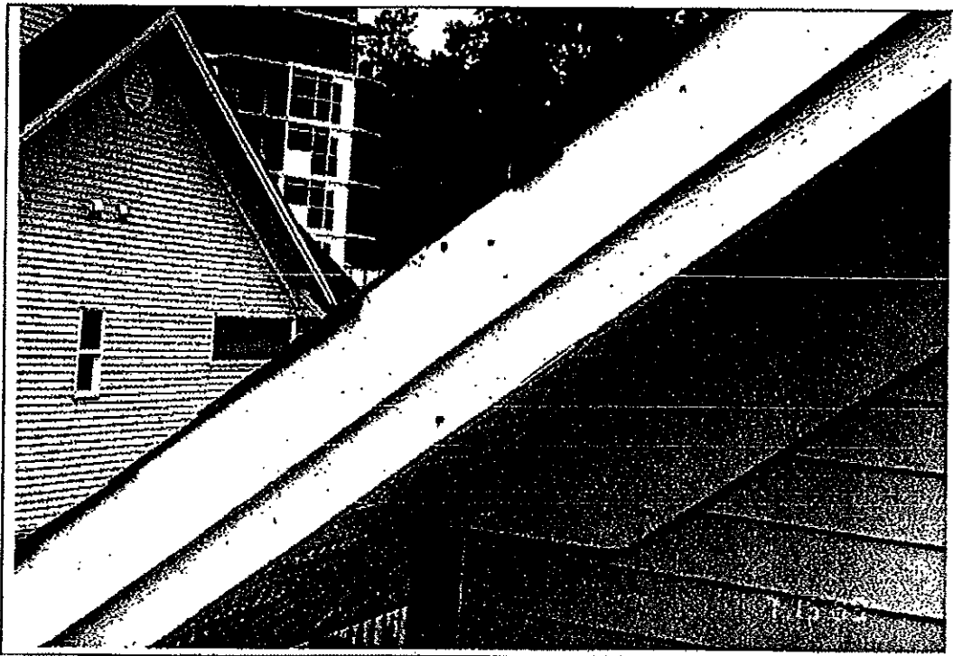
Photo No. 30 – Location where satellite dish had been secured to the roof fascia board above unit 65.
