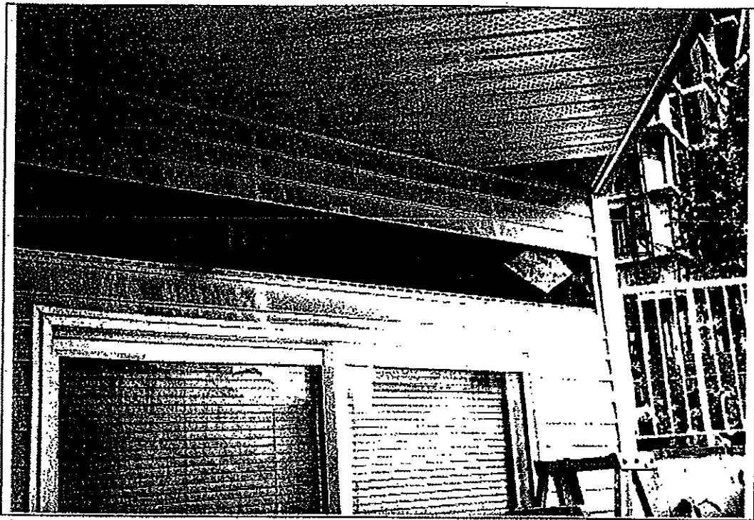
Photo No. 17 – Exploratory opening no. 6, revealing the OSB sheathing and gypsum soffit sheathing to be in reasonable condition.
