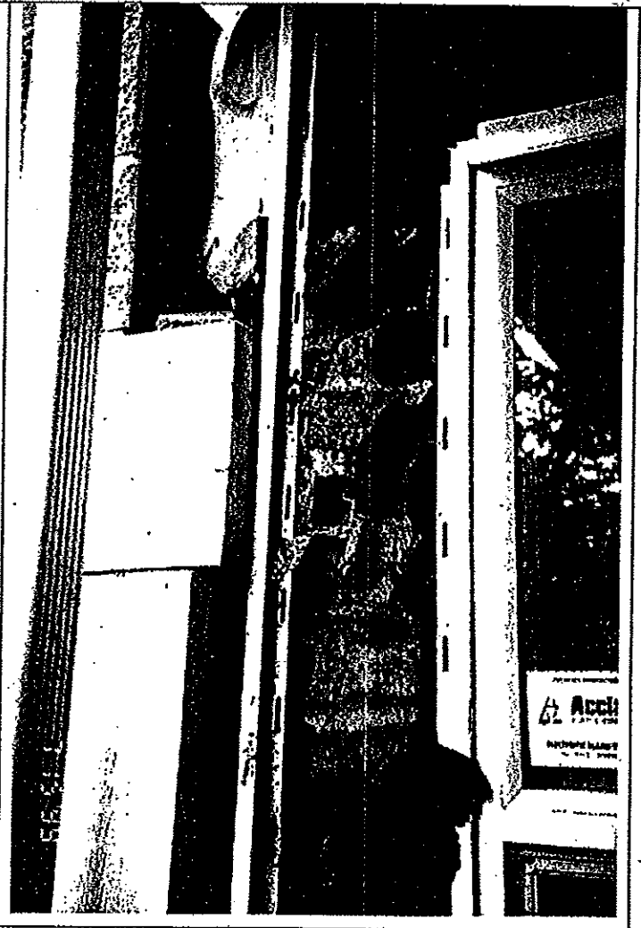
Photo No. 14 – Exploratory opening no. 3 (close-up), revealing the deterioration of the building paper and gypsum sheathing.
