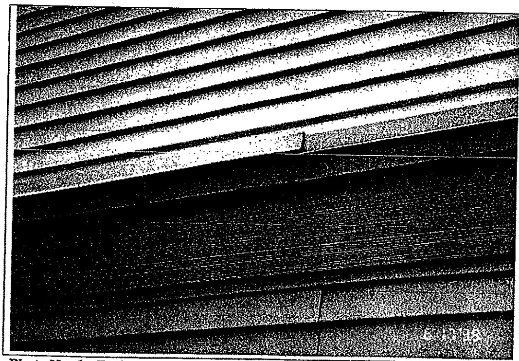
Photo No. 6 – Typical unsealed lap in the metal flashing over the wood bands at floor levels.
