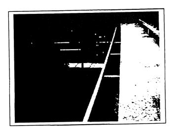
Photo 10 Some balconies drain off the edge into gutters. These gutters should be inspected and cleaned once per year or as required.
