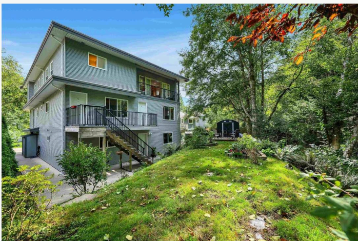
Rear elevation — independent suite entries and exterior stair
