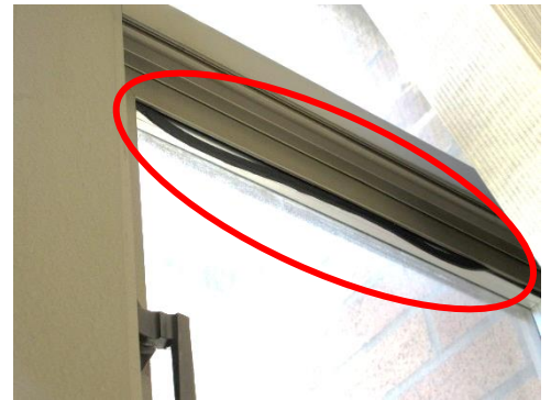
Photo 21: Interior glazing sagging out of window frame.
