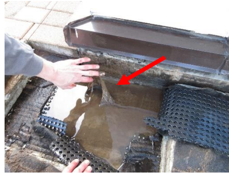
Photo 33: Ponding water and deteriorate membrane at roof opening at PH-1 upper roof deck
