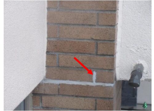
Photo 48: Caulked weep hole at brick veneer cladding.
