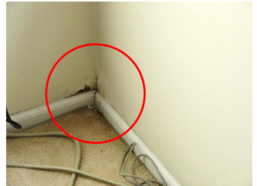
Photo 11: Damaged and moist drywall below window at Suite 1903.
