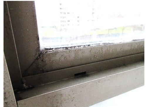
Photo 19: Condensation on window framing.
