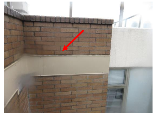
Photo 49: Wall flashing over brick veneer cladding.
