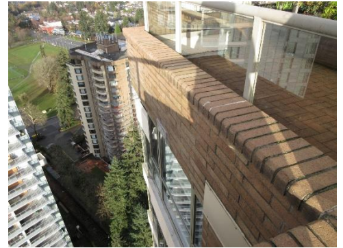
Photo 50: Brick clad parapet wall at penthouse roof deck.
