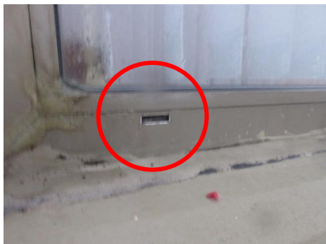
Photo 16: Typical exterior window drain hole at window sill.
