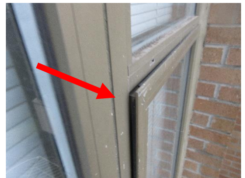
Photo 18: Operable windows not closing tightly.
