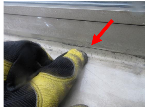
Photo 13: Debonding caulking at window sill.
