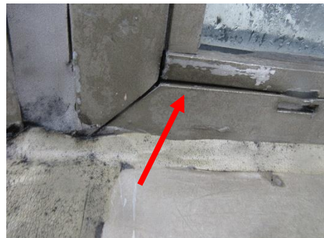
Photo 15: Gaps between window frame and exterior glazing stop.
