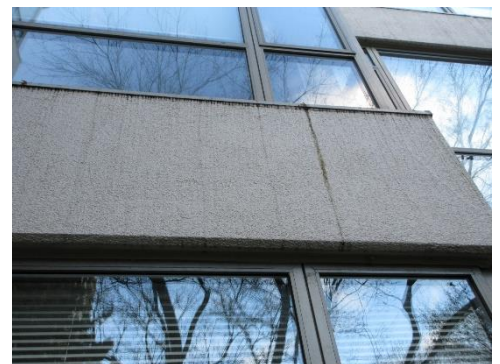
Photo 43: Typical concrete curb wall.
