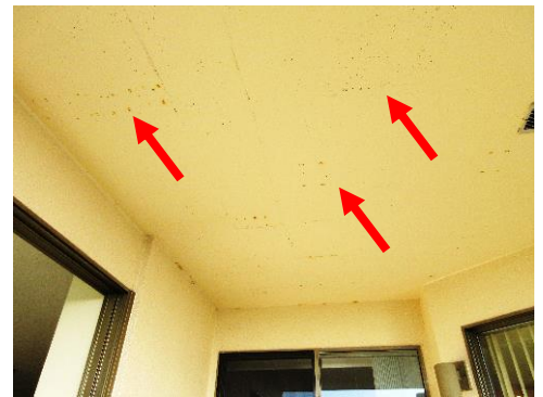
Photo 42: Rebar staining on soffits.
