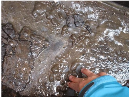
Photo 34: Waterproofing membrane with blisters at PH-6 roof deck.
