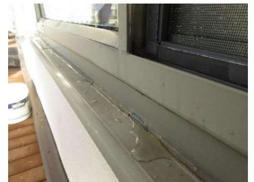
Photo 51: Back-sloped balcony flashings.
