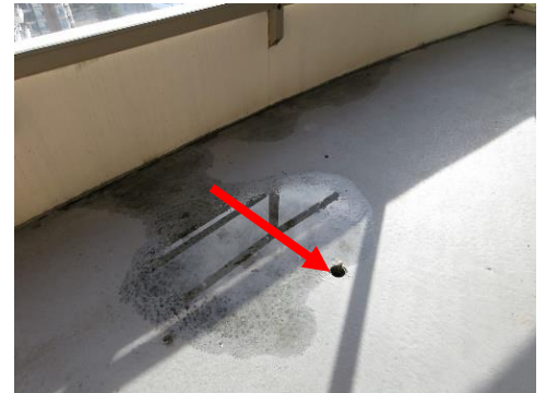
Photo 41: Missing balcony drain cover.
