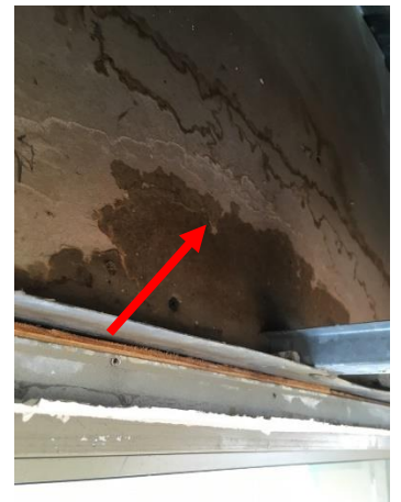
Photo 28: Water stain above PH-1 sliding door head, roof soffit space.
