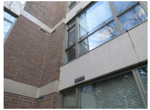
Photo 44: Typical brick veneer clad wall.
