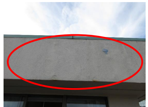
Photo 47: Blistered stucco at the main sloped roof parapet wall.
