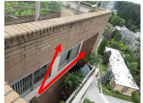
Photo 30: Brick cladding column and unprotected brick on a horizontal surface
