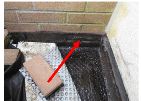
Photo 31: Waterproofing membrane upturns onto the outside surface of the brick cladding.
