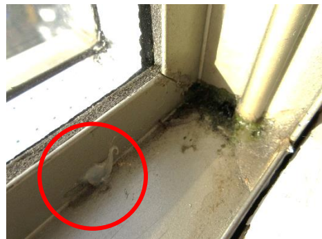
Photo 17: Interior drain hole filled with caulking.
