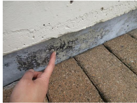
Photo 35: Flaked/peeled waterproofing membrane at PH-3 roof deck parapet wall
