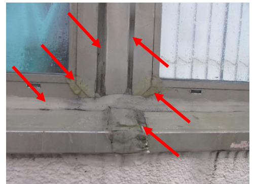
Photo 12: Typical window with varying caulking at exterior at North Elevation.
