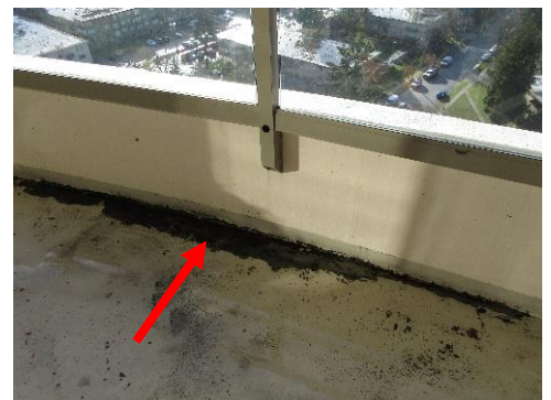
Photo 40: Failed balcony waterproofing membrane.
