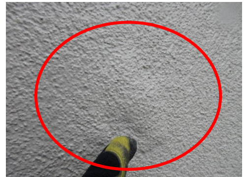
Photo 46: Blistered acrylic coating on concrete wall.
