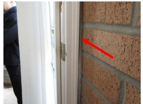
Photo 23: Wood door frame to brick cladding joint not caulked.
