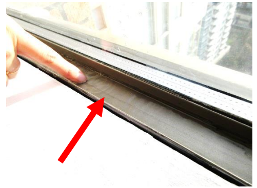
Photo 10: Pooling water in window track at PH-05.
