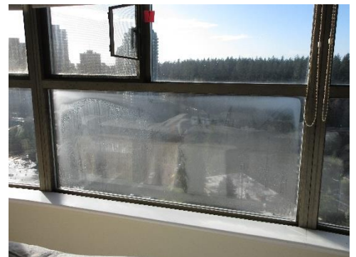
Photo 20: Typical failed IGU.
