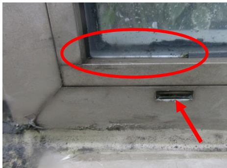
Photo 14: Shrunk/missing exterior glazing gasket at window sill and drain hole with visible water sitting in framing (arrow).
