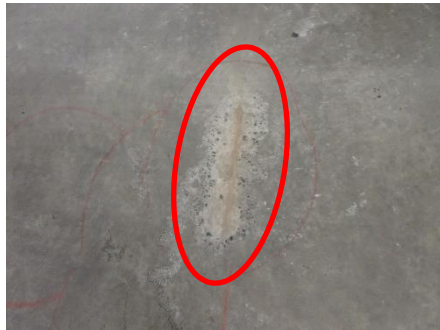
Photo 15: Typical topside delamination with exposed reinforcing steel.
