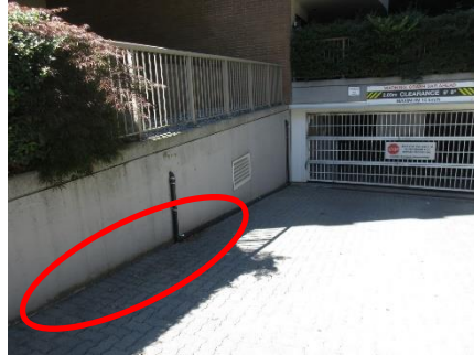
Photo 6: Entrance leaking entrance ramp to wall joint.
