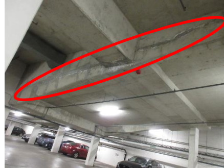
Photo 7: Entrance ramp staining along bottom of wall.
