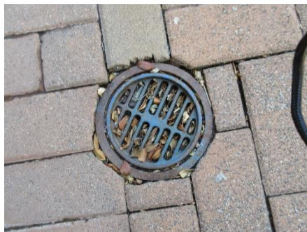
Photo 4: Plugged walk-way drain at north-west side, next to pool area.
