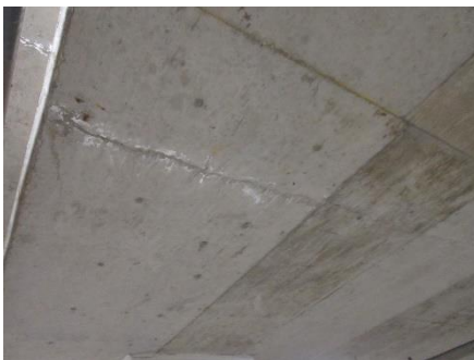
Photo 10: Efflorescence on soffit of suspended slab.
