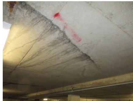
Photo 3: Cracks with evidence of leakage on garage soffit.
