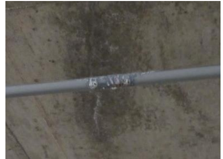
Photo 19: Typical corrosion on sprinkler pipes.
