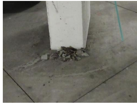
Photo 14: Loose concrete that has fallen from soffits during concrete sounding that was completed during the garage evaluation.
