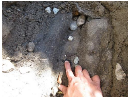
Photo 2: Moisture below garage roof waterproofing.
