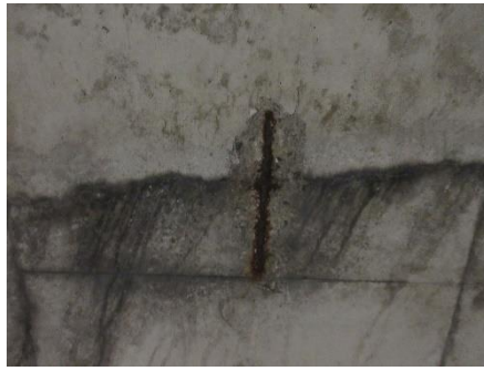
Photo 13: Typical exposed reinforcing at concrete spall location.
