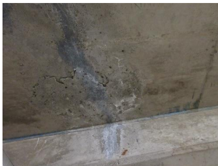
Photo 11: Typical delaminated concrete on suspended slab soffit.
