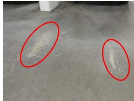
Photo 16: Typical topside delamination with exposed reinforcing steel.
