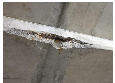
Photo 12: Loose concrete broken off when concrete sounding was completed during the garage evaluation.
