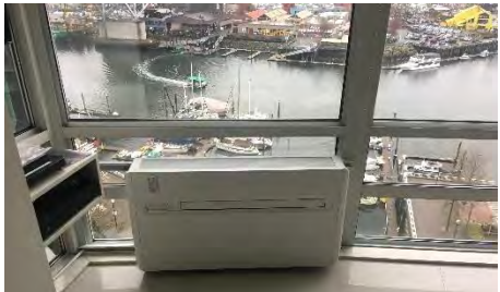
Photo 4: Example of interior contained heat pump.
