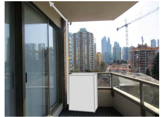
Photo 5: Typical balcony location for outdoor unit and lines connecting indoor and outdoor units.
