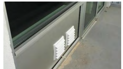
Photo 6: Exterior of an interior contained heat pump penetrating a metal panel below a window.
