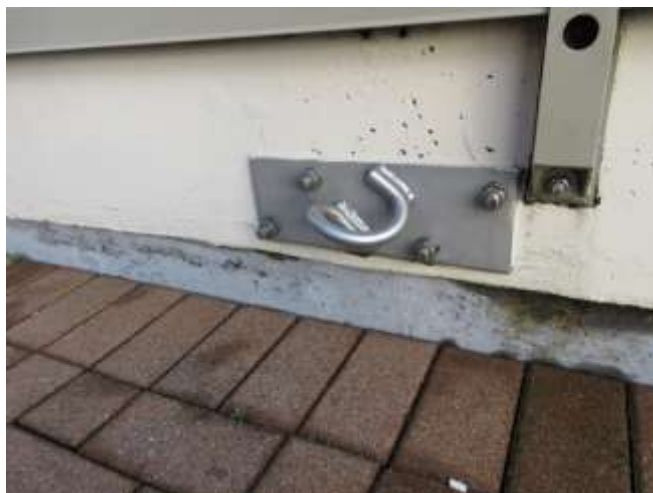
Photo 3: Typical adhesive wall anchor.
