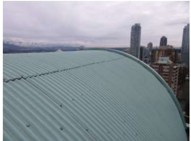
Photo 8: Sloped metal roofing.
