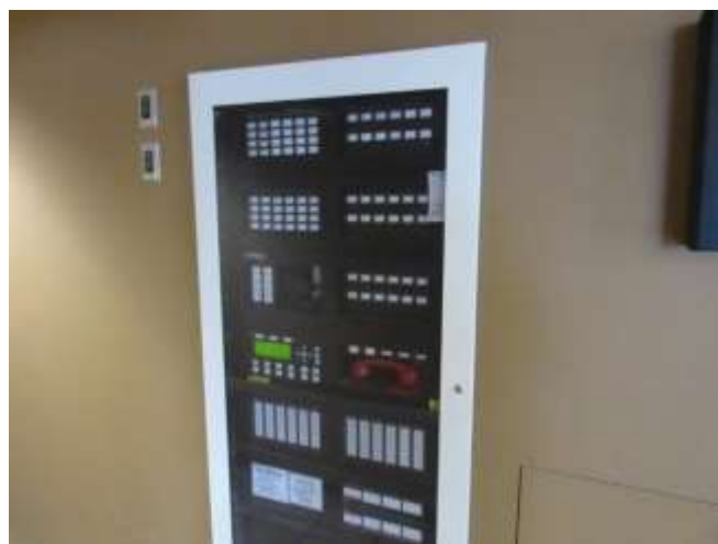
Photo 10: Fire alarm control panel.
