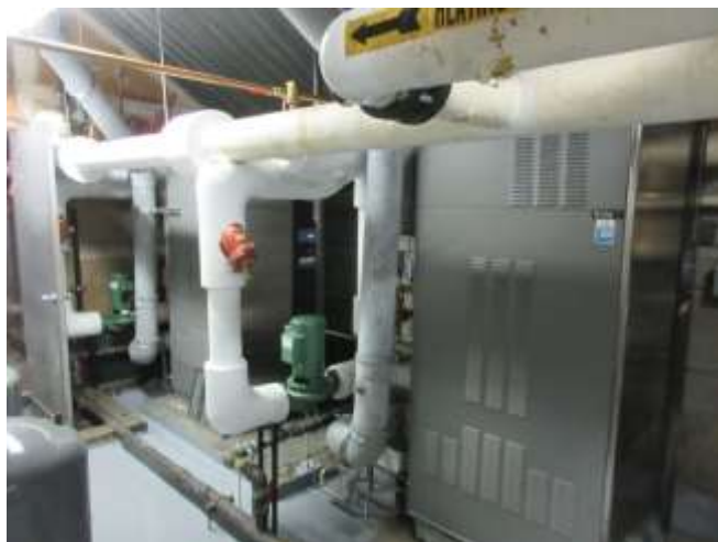
Photo 16: Hydronic heating boilers.
