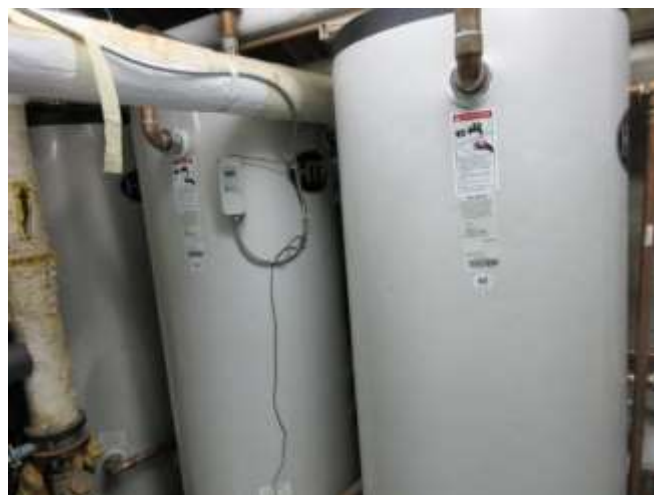
Photo 19: Domestic hot water storage tanks.
