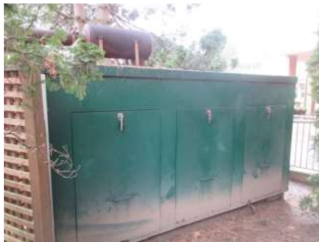
Photo 12: Emergency generator enclosure.
