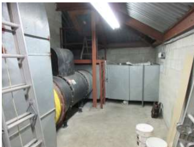
Photo 17: Roof-top air handling unit and supply fan.
