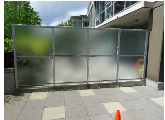
Dividing wall on patio
