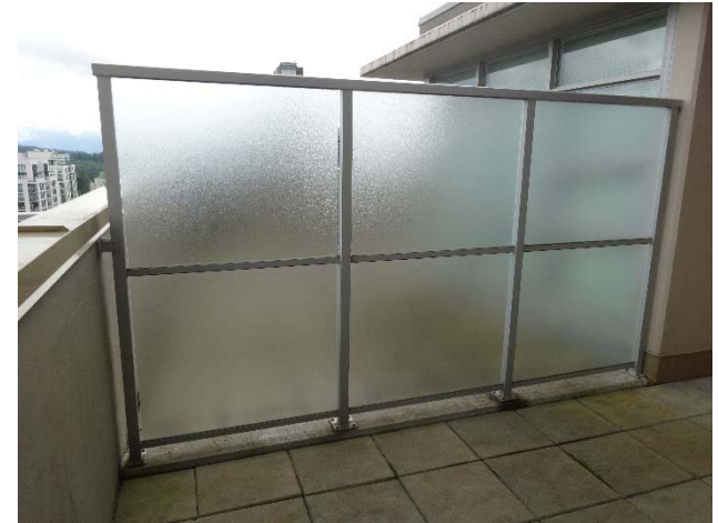
Dividing wall on roof terrace
