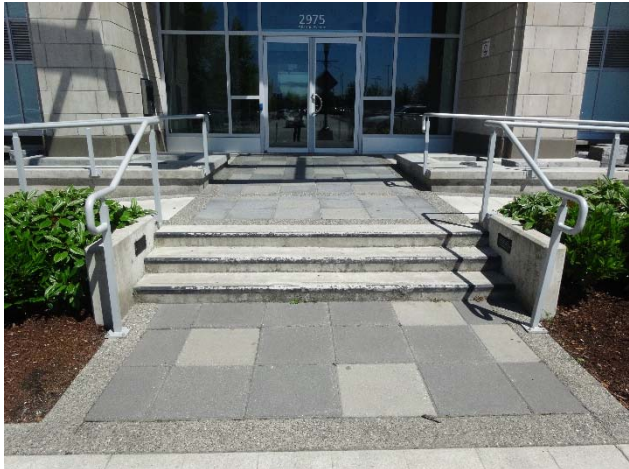
Exterior stairs with railings
