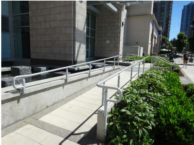
Ramp with railings
