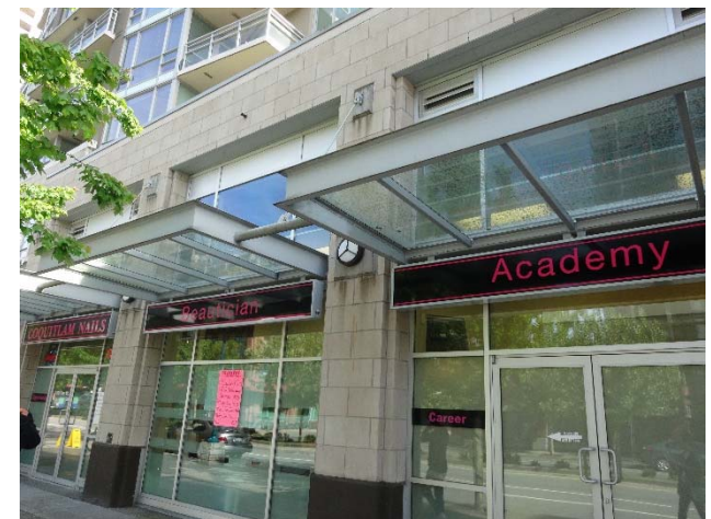
Storefront windows – commercial units
