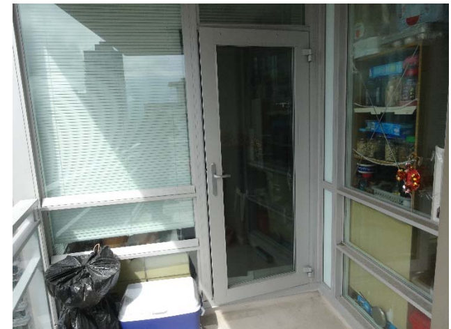
Swinging door on balcony
