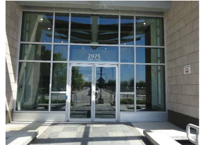
Main entrance door
