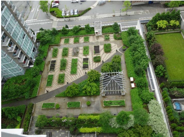
Areas with waterproofing membrane
