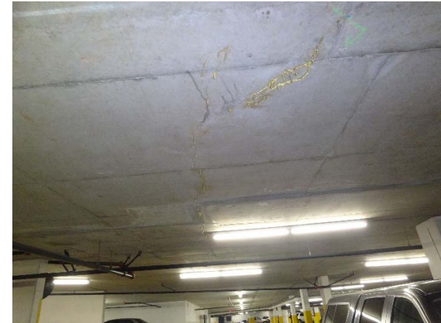
Light fixture in parkade
