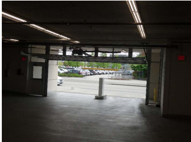
Concrete pavement in front of garage entrance
