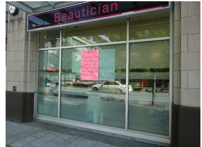
Storefront windows – commercial units
