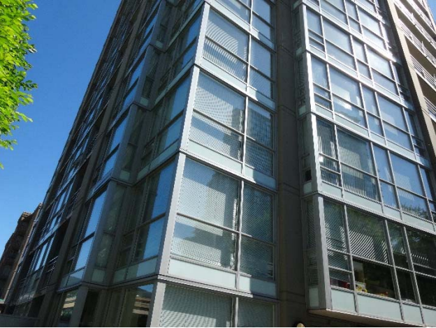
Exterior windows - residential
