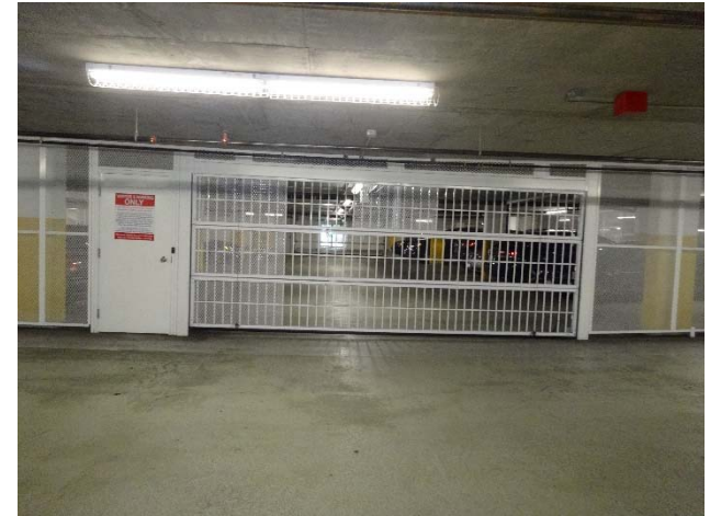
Interior garage door
