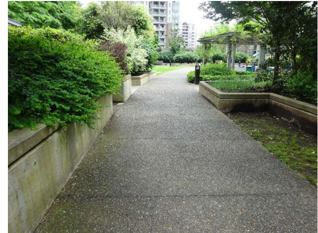
Pedestrian walkway on roof top garden
