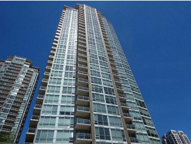
Exterior windows - residential
