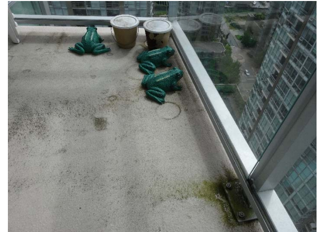
Liquid membrane on balcony decks
