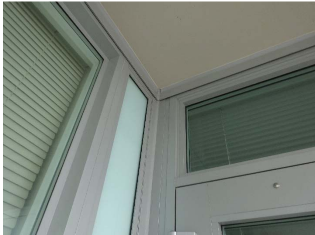
Caulking between door/windows frames and ceiling
