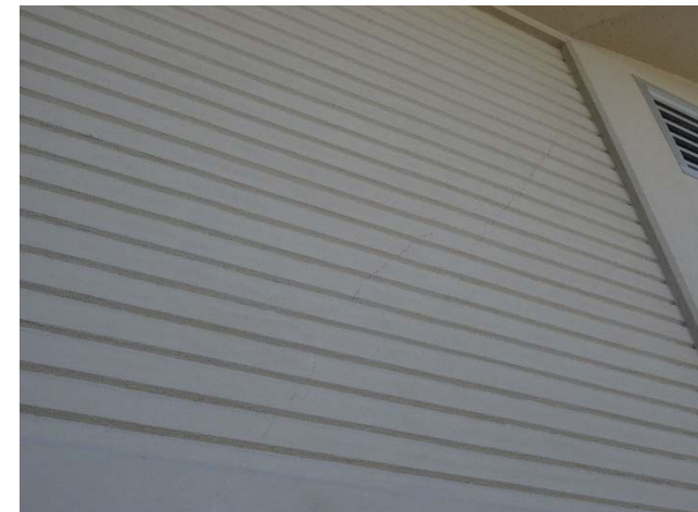
Diagonal crack
