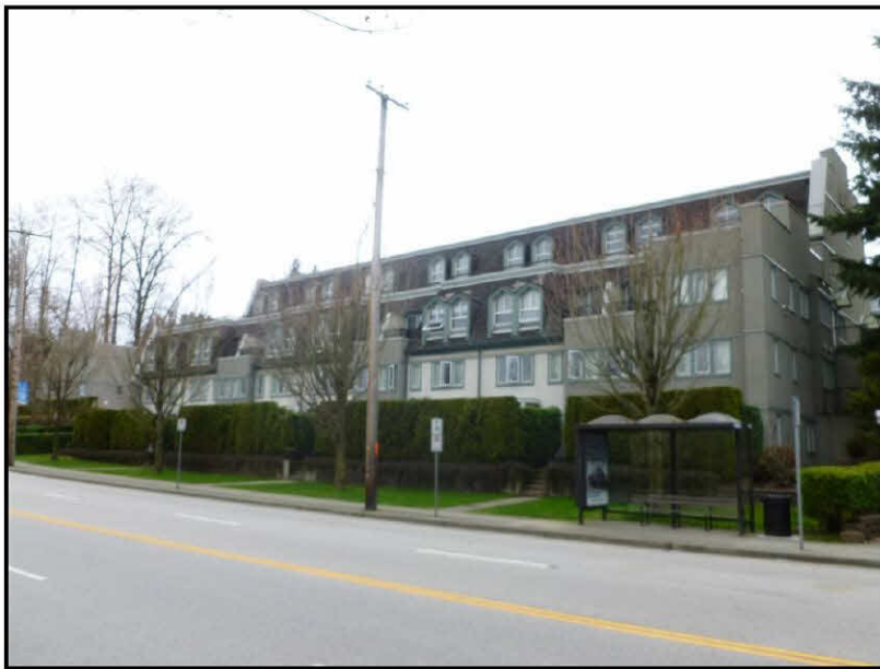
Photo No. 2: South elevation of Building E
