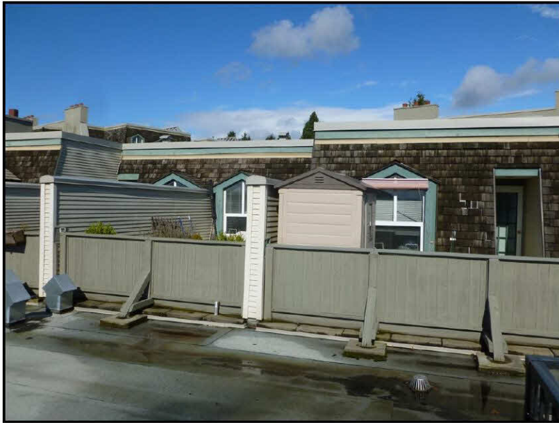
Photo No. 17: Typical third floor small terrace
