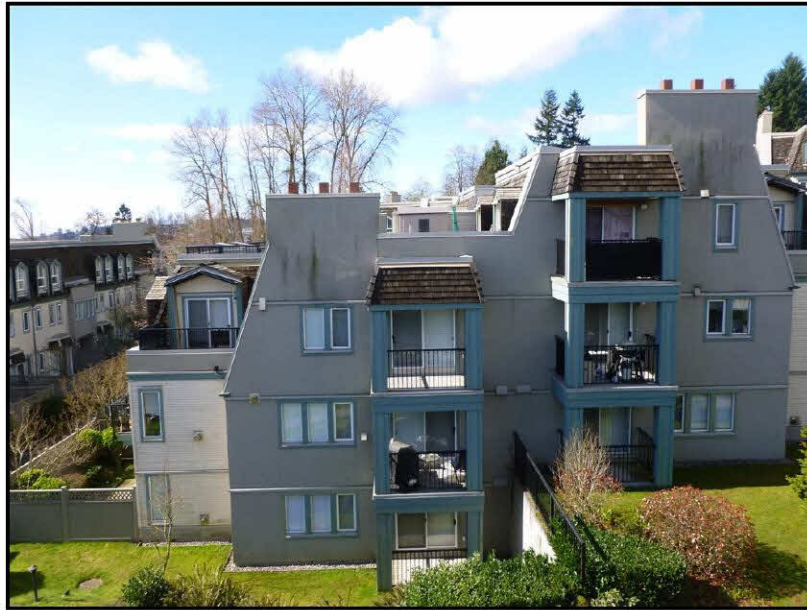
Photo No. 7: East elevation of Building D
