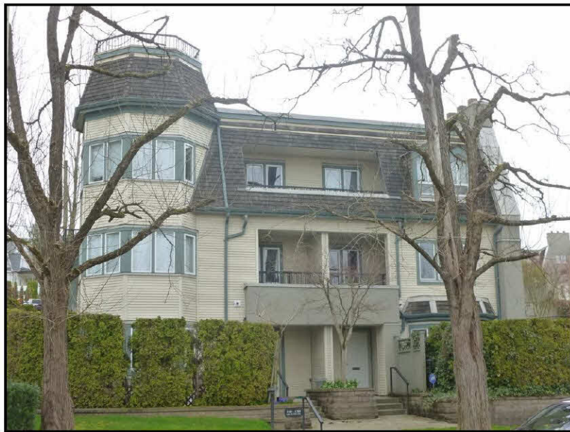
Photo No. 8: South elevation of The Gatehouse
