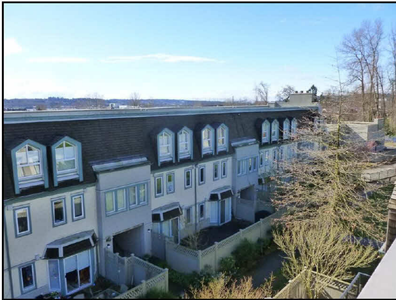
Photo No. 4: North elevation of Building E
