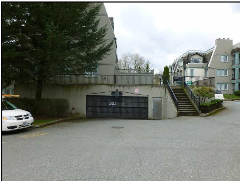
Photo No. 18: Entrance for Garage 5
