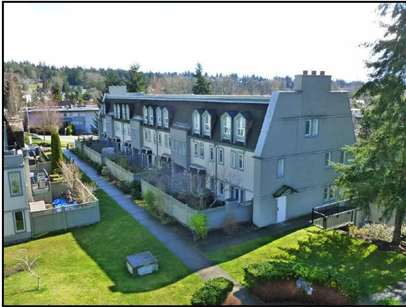
Photo No. 5: North elevation of Building F
