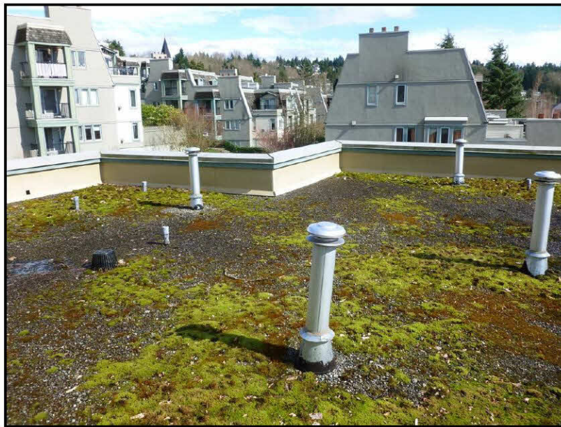
Photo No. 14: Built-up roof for The Gatehouse
