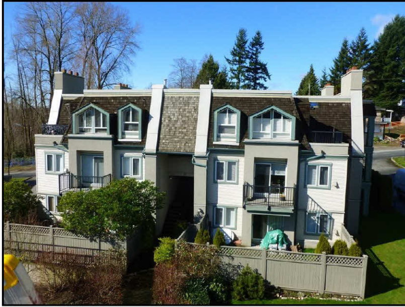
Photo No. 3: East elevation of Building C
