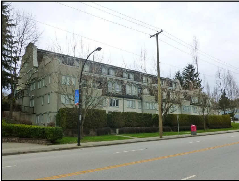
Photo No. 1: South elevation of Building F
