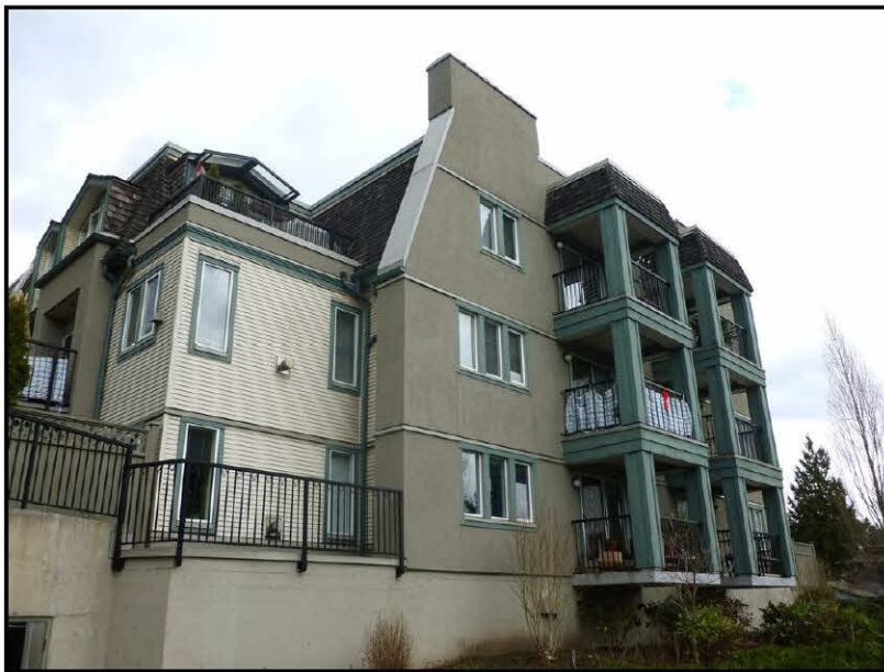
Photo No. 6: South elevation of Building H
