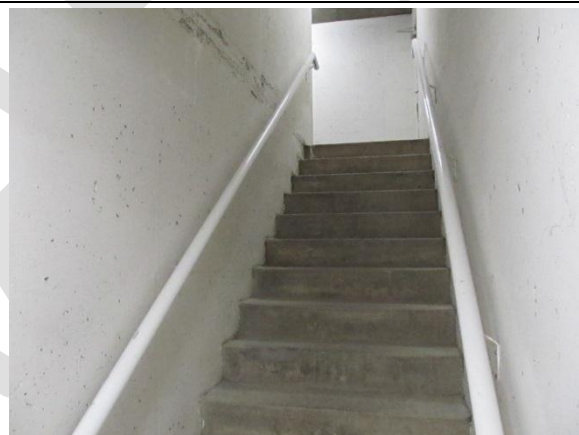
Typical painted concrete stairwell.
