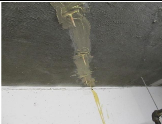
Epoxy-filled cracks on underside of at-grade concrete suspended slab.
