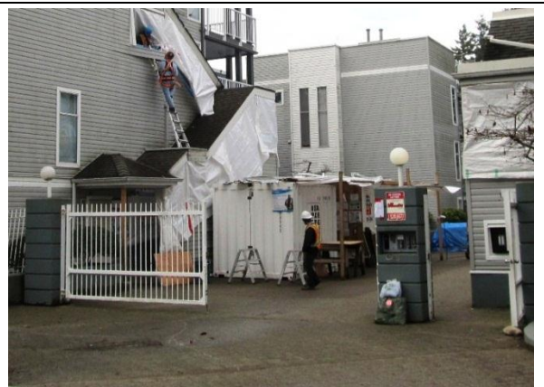
Illumination at pedestrian entrance.
