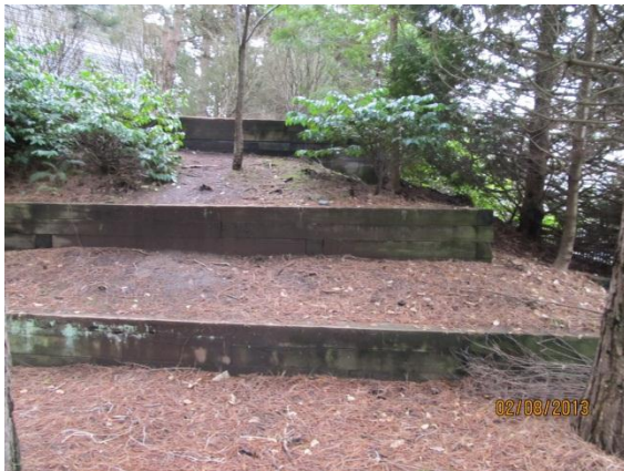
Stepped timber retaining walls in northwest yard.
