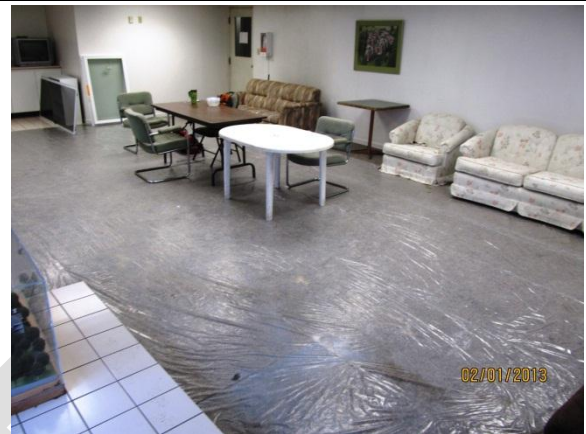
Protective plastic covered existing carpet in Community Room during room repairs.
