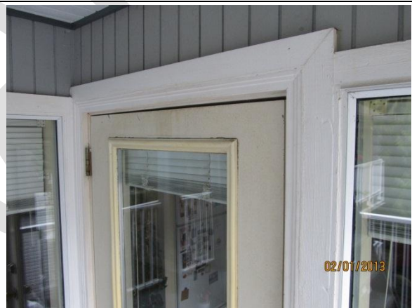
Typical wood board-sided balcony walls.
