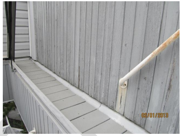
Typical interior side of roof deck guardwall.
