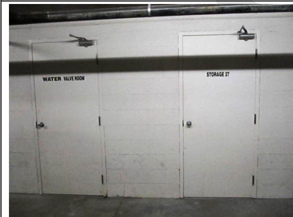
Painted concrete wall at storage lockers.
