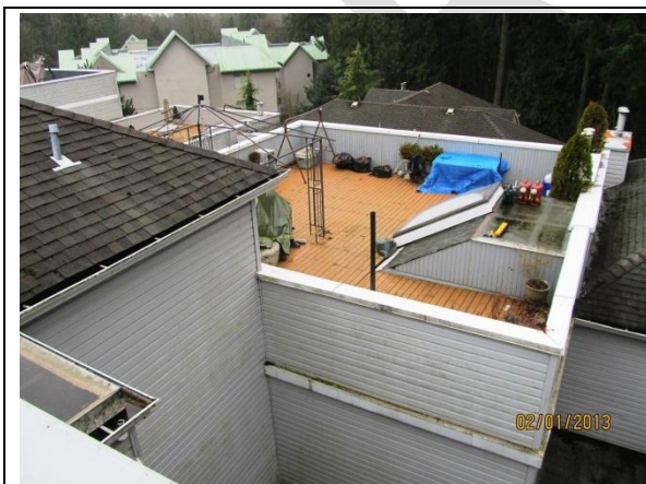
Typical roof deck.
