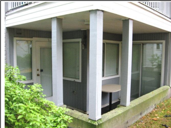
Typical wood board-sided patio walls.
