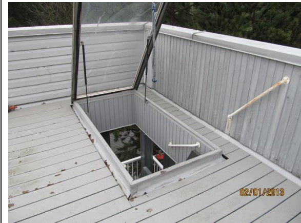
Typical roof deck.
