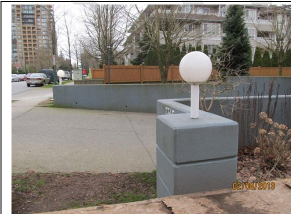
Illumination at vehicle entrance.
