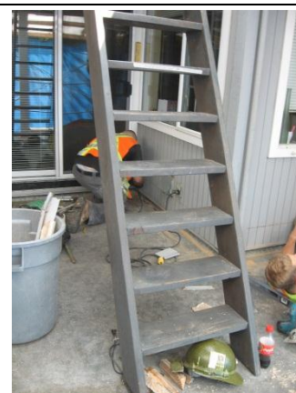
Wood-framed ladder-stairs to typical roof deck.
