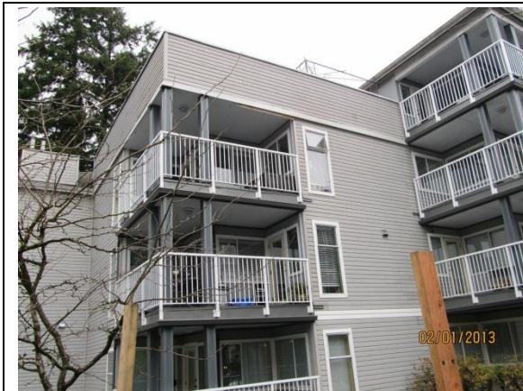
Typical stacked balconies.
