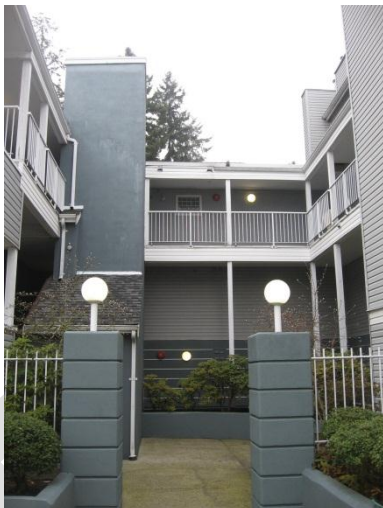
Stucco cladding on elevator shaft wall.
