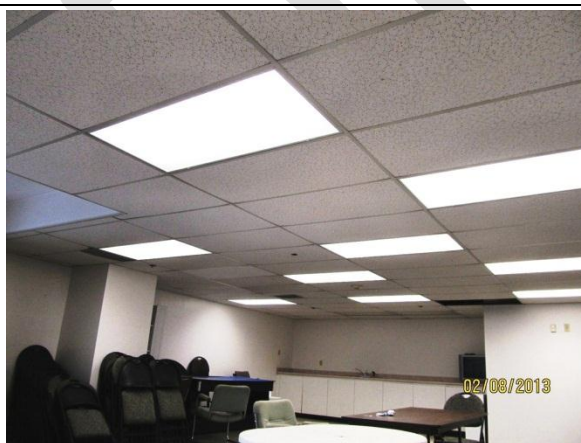
Suspended ceiling with acoustic panels.
