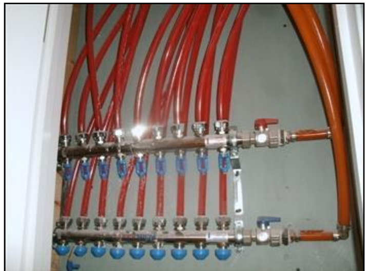
Left side of basement: for the 1st floor.
