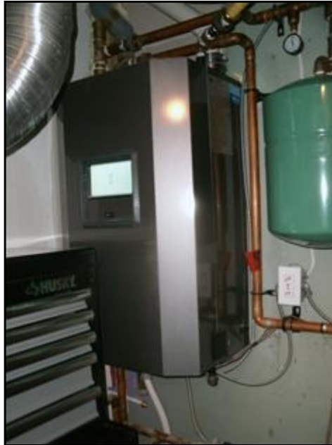
Boiler (hot water): On-demand water heater
