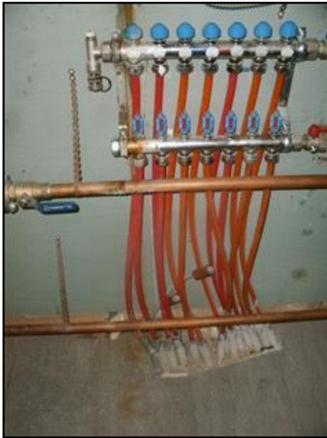
Going into basement slab
