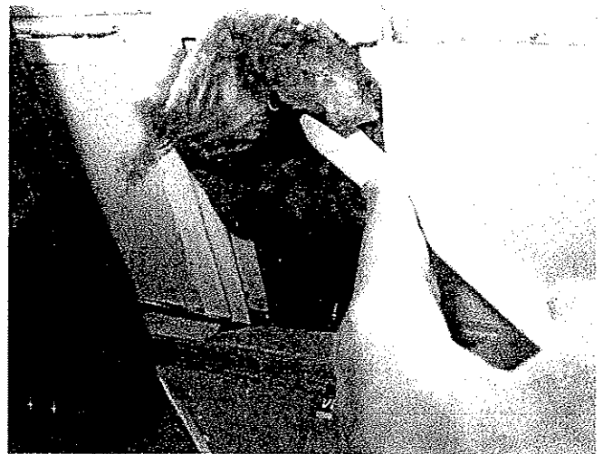
415 Moisture ingress within window wall assembly at
