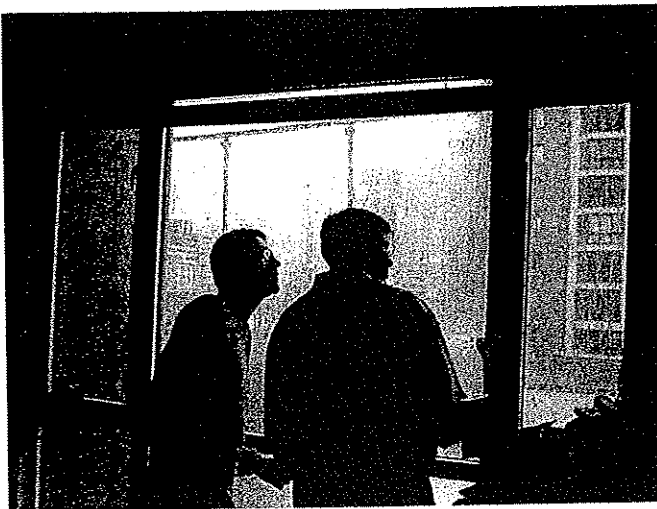
406 Window test #1 at window wall, unit 605
