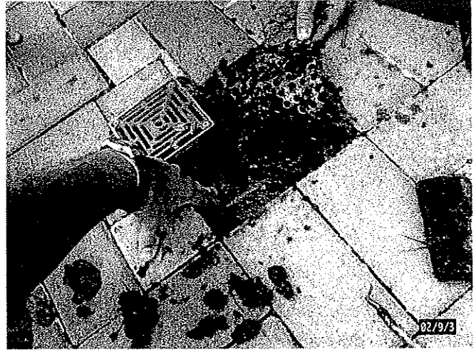
932 Hot rubberized membrane and sheet membrane
