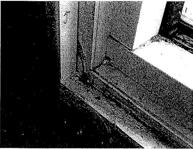
408 Water ingress at window frame, test #1
