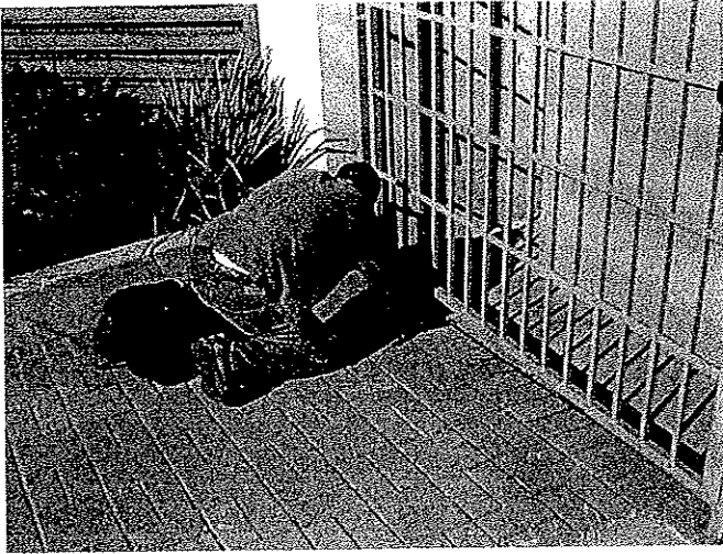
923 Paver removal for membrane examination, north
