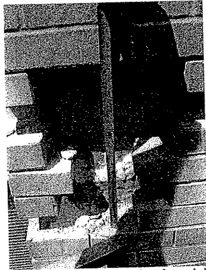
501 1608 brick removal, no ties for minimum 28
