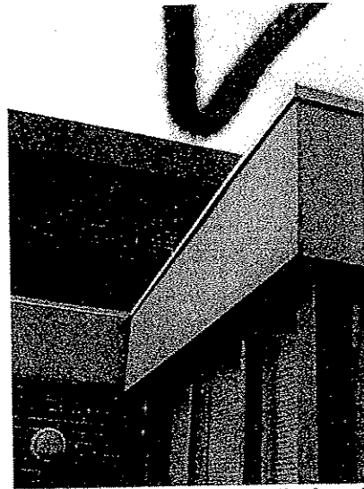
901 EIFS band at window wall of roof deck
