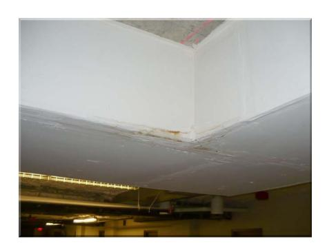
PHOTO M-22 Leak in parkade drywall bulkhead.
