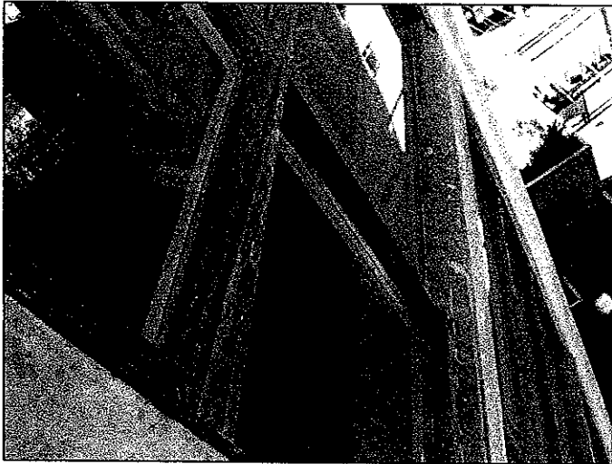
Photo #25- Concrete splashed on window frames.
