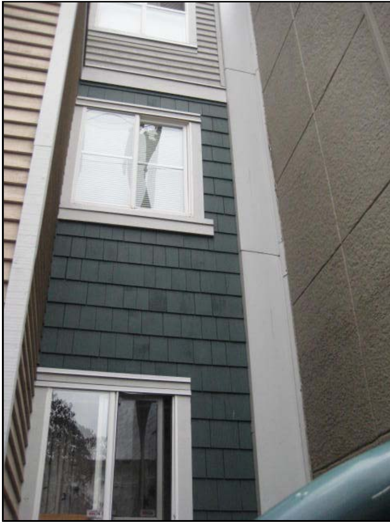
Photo No. 6: West Elevation, Painted Wood Shingles
