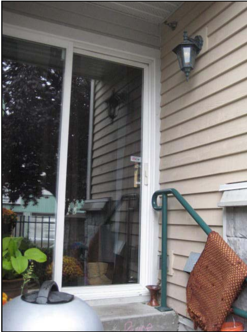
Photo No. 11: Typical Patio Entrance at West Elevation
