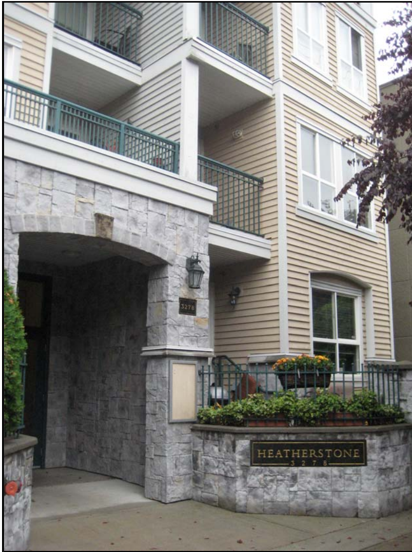
Photo No. 1: Front Entrance, West Elevation
