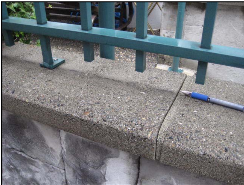
Photo No. 16: Perimeter Site Wall
