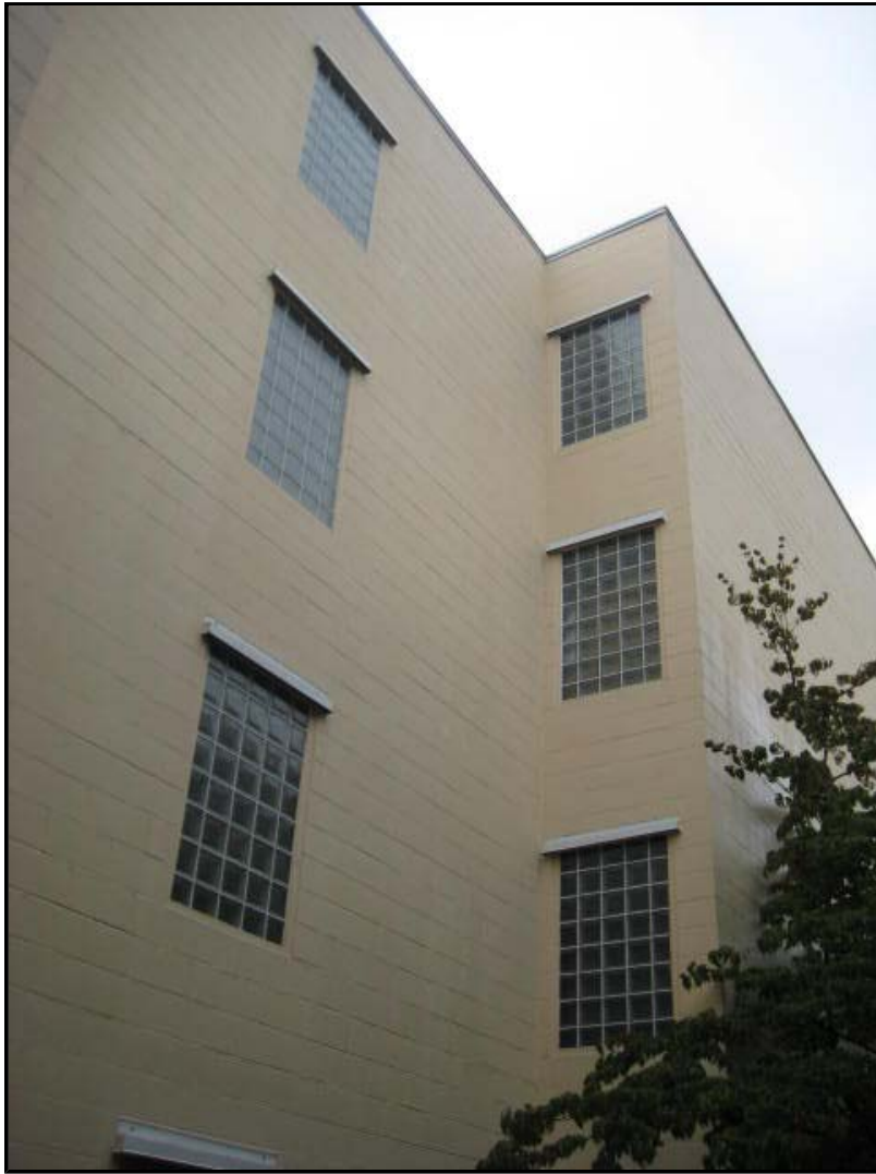
Photo No. 3: South End Wall
