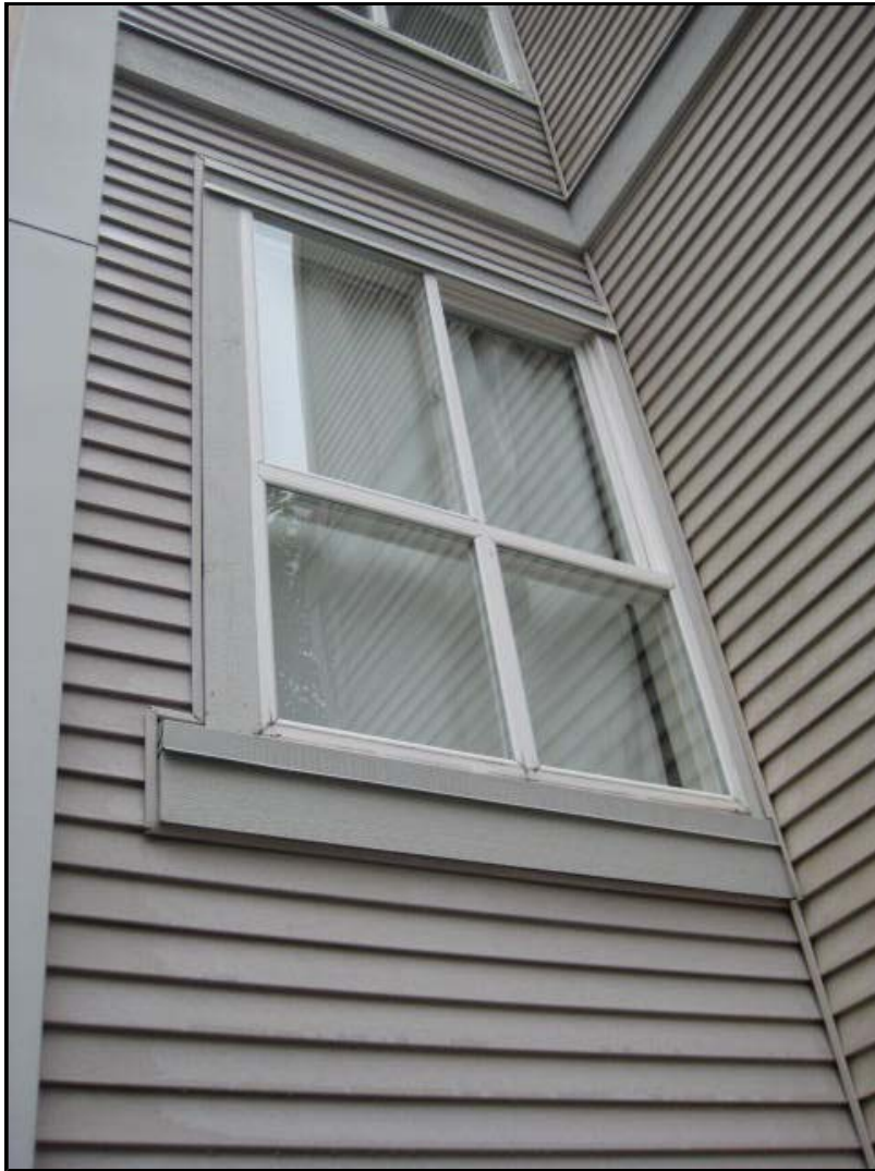
Photo No. 8: Typical Window Note: Wood trim and metal drip flashings.
