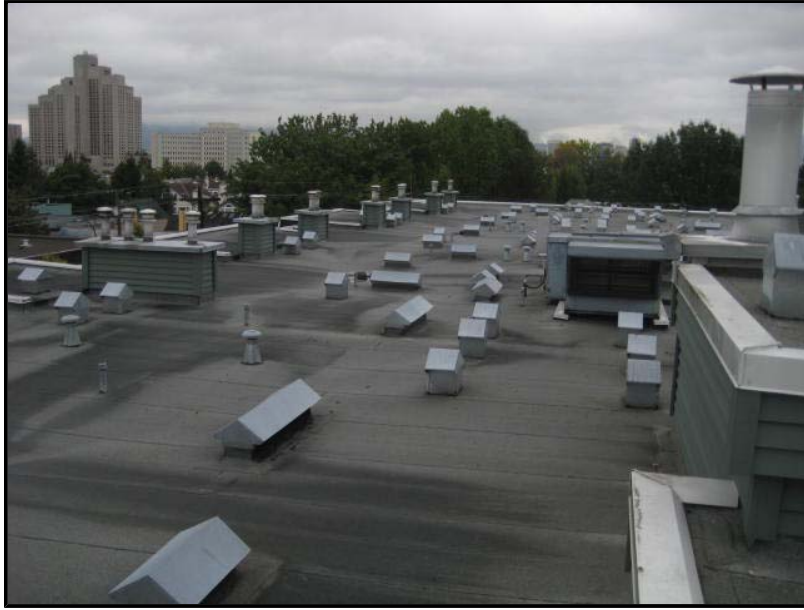
Photo No. 12: Roof
