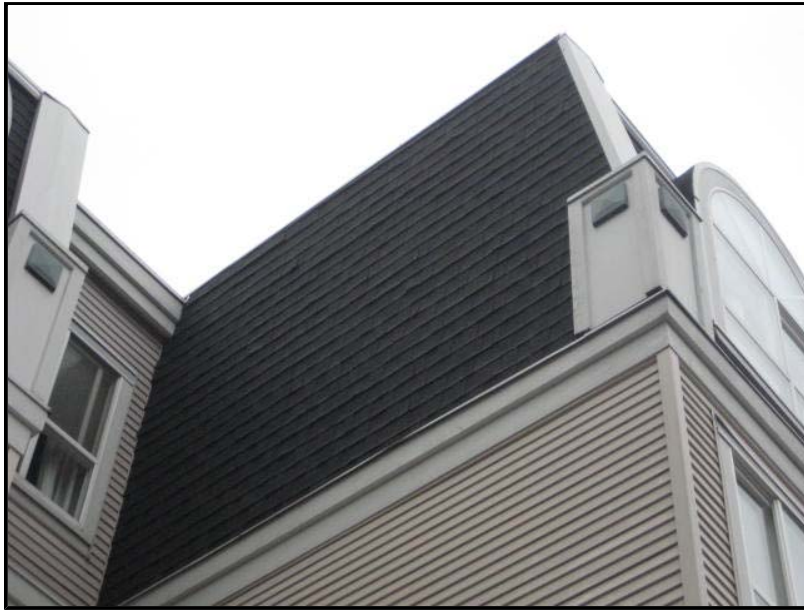
Photo No. 7: Typical Mansard Roof
