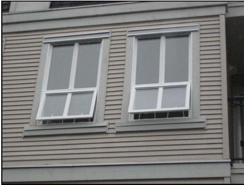
Photo No. 9: Replacement Fixed Over Awning Style Windows
