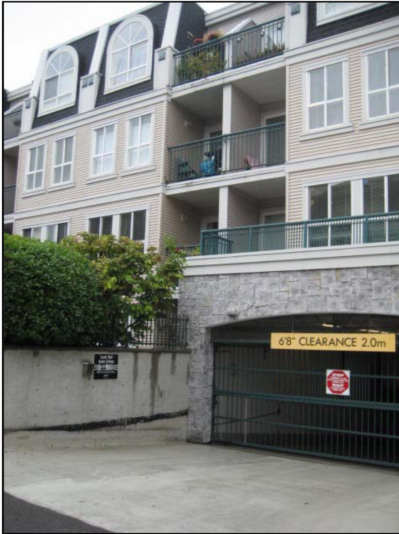
Photo No. 2: East Elevation, Garage Entrance
