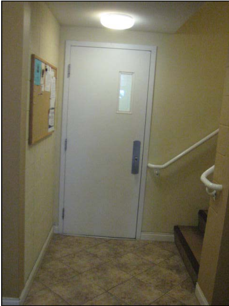
Photo No. 14: Typical Stairwell
