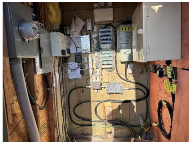
Photo 42. Interior view of the front entrance gate house.
