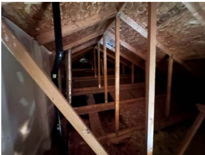
Photo 5. Example view of an attic space at a townhouse unit.
