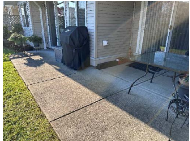
Photo 44. Example view of the concrete patio.
