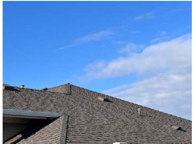
Photo 28. Another view of the asphalt shingle roof.
