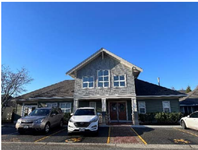
Photo 17. Front elevation of the Amenity Building.
