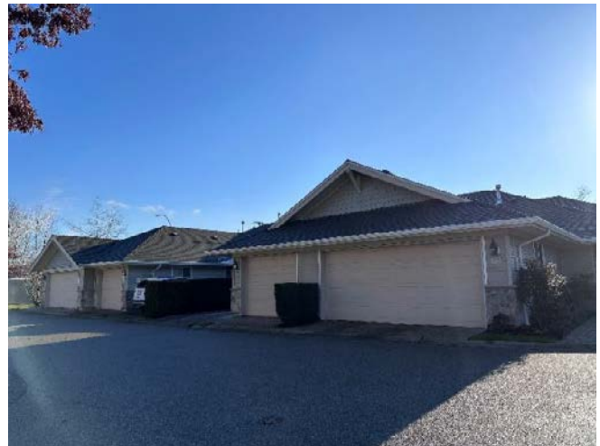
Photo 30. Front elevation view of a three-plex townhouse block.
