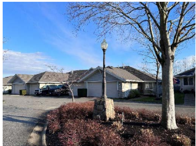
Photo 24. Example view of a light standard at the roadway.
