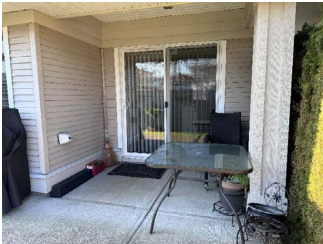
Photo 45. Example view of the sliding glass door.
