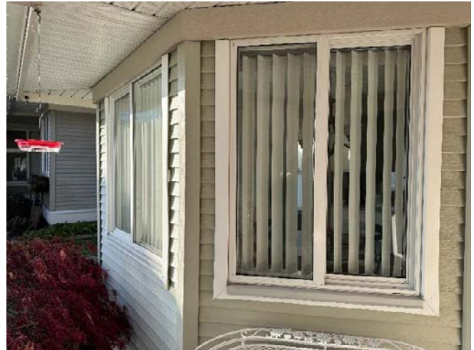
Photo 2. Example view of a window assembly.
