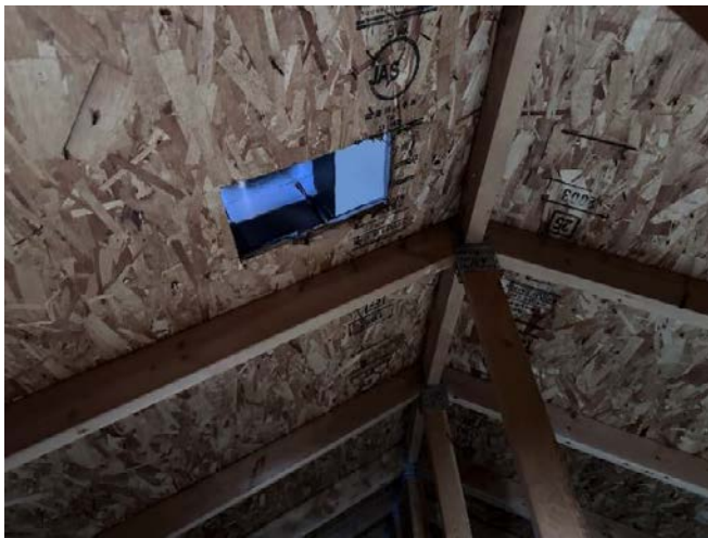
Photo 3. View of the attic sheathing and roof vent.
