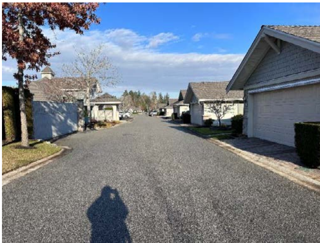
Photo 21. Overall view of the asphalt paved roadway at the property.
