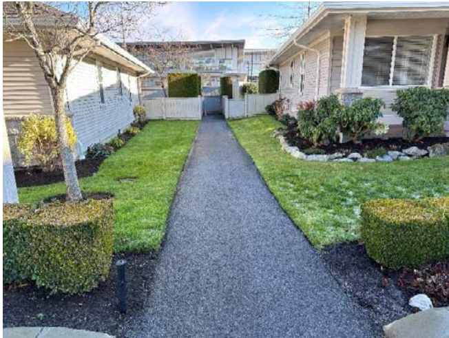
Photo 37. Example view of the asphalt paved walkway.
