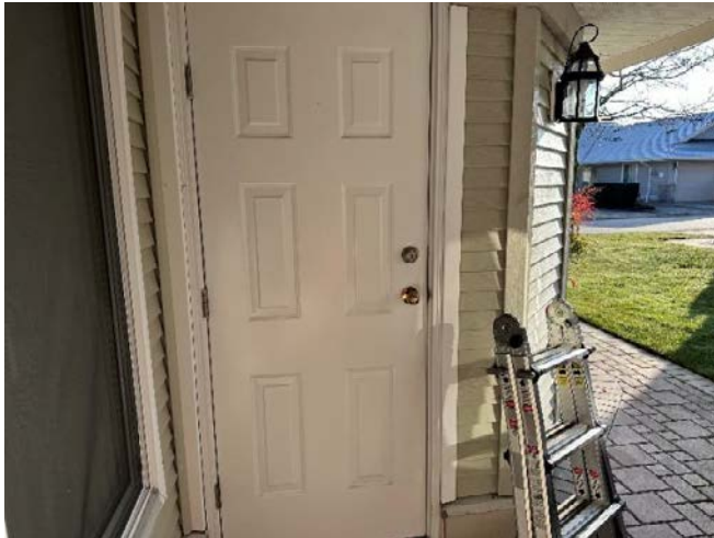
Photo 1. Example view of a man-door into a garage.
