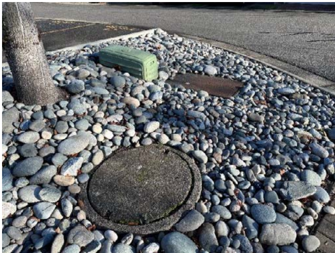
Photo 35. View of the utility boxes and storm drain at the property.
