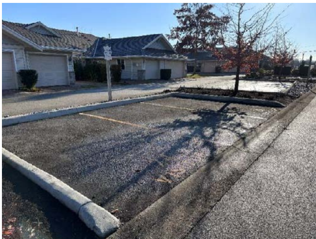
Photo 23. Parking stalls located along the roadway.
