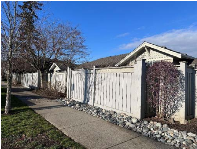
Photo 27. Example view of the wood fencing at the east perimeter of the property.
