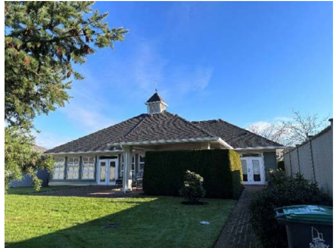
Photo 20. Rear elevation of the Amenity Building.
