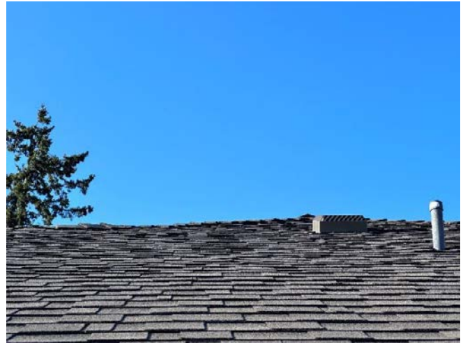
Photo 26. Example view of the asphalt shingles at an upper sloped roof.
