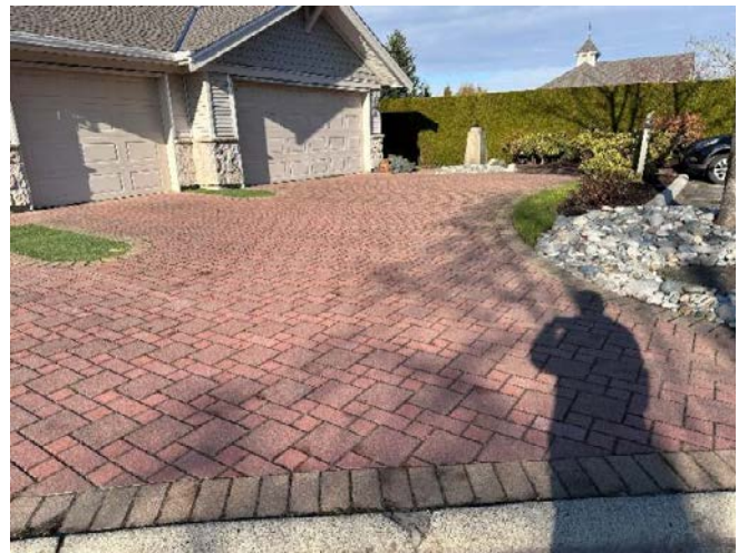
Photo 22. Example view of the paving stone at the property.
