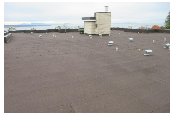
SBS membrane roofing
