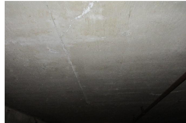
Parkade roof deck
