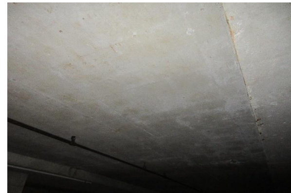
Parkade roof deck
