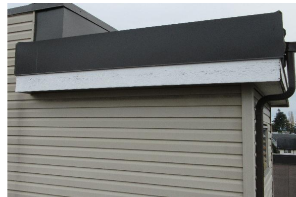
Exterior wooden fascia board
