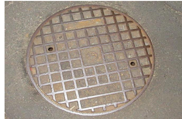
Sanitary manhole cover
