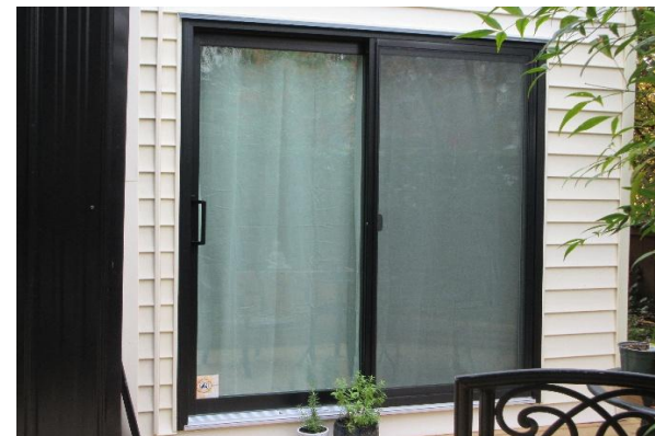
Aluminum slider doors with tempered glass
