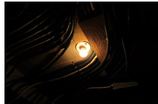
Service room light fixture
