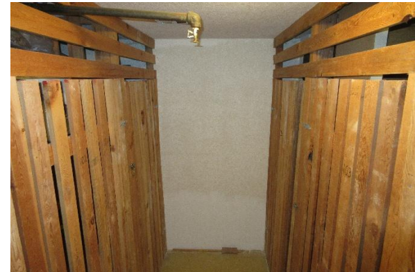
Storage room finishes
