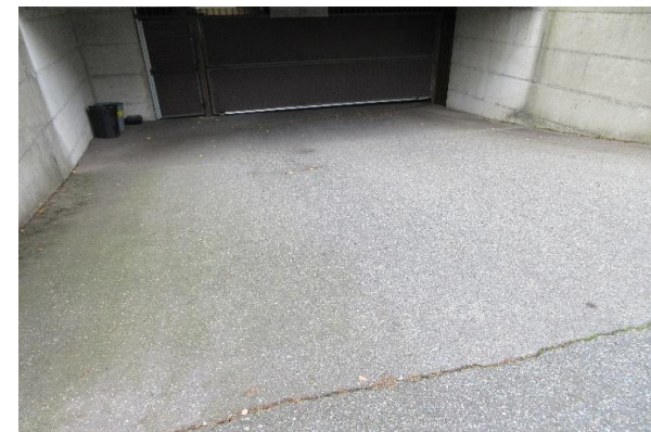
Exterior concrete paving
