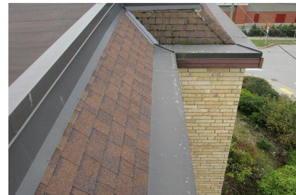
Asphalt shingle roofing
