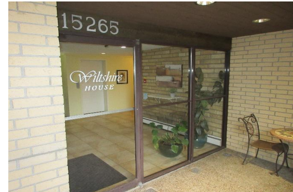
Aluminum glass swinging main entrance door
