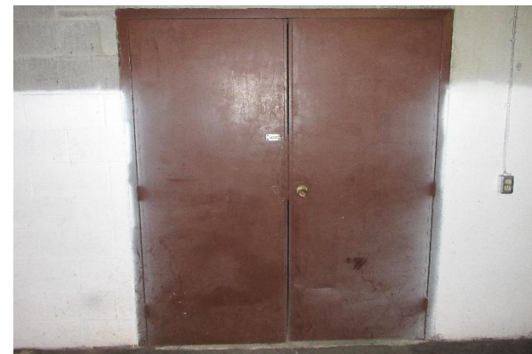
Metal service doors
