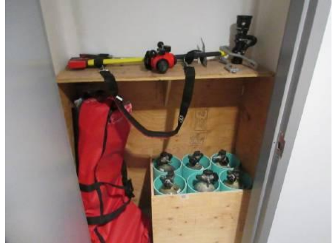
Photo 15: Typical firefighter's closet.
