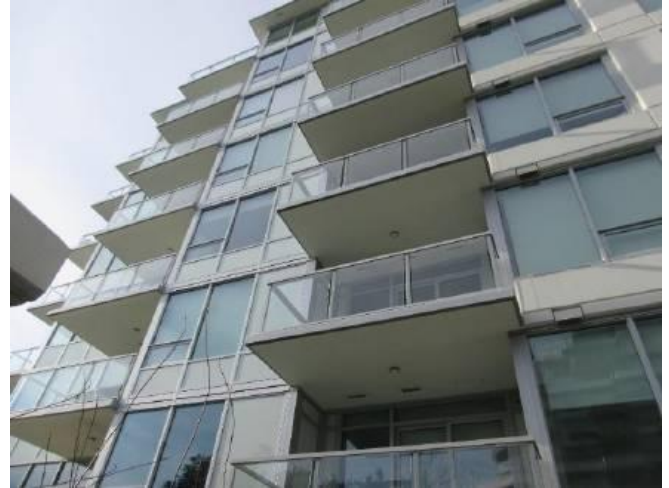
Photo 4: Typical tower balconies.
