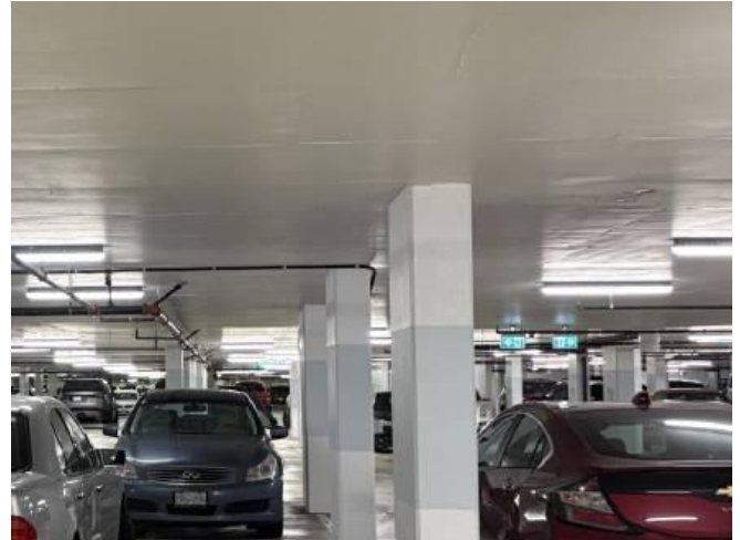
Photo 1: Typical structure in the parking garage.
