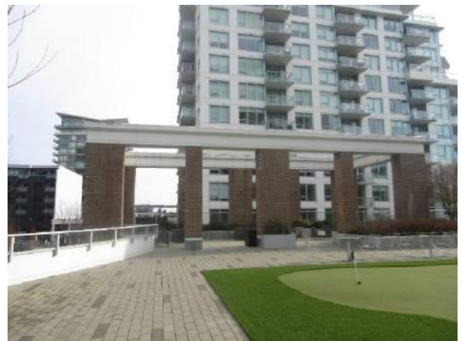
Photo 2: Brick-clad pergola structure.
