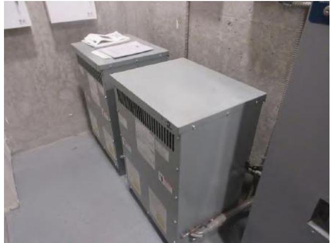
Photo 41: Typical machine-room-less elevator equipment.
