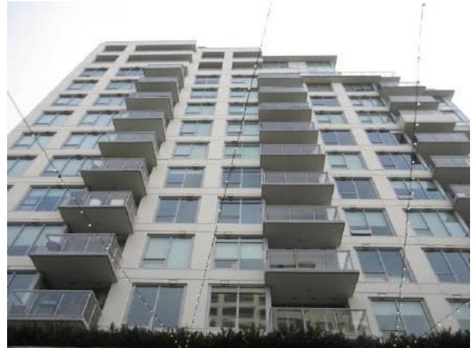
Photo 8: Typical exterior walls at the towers.
