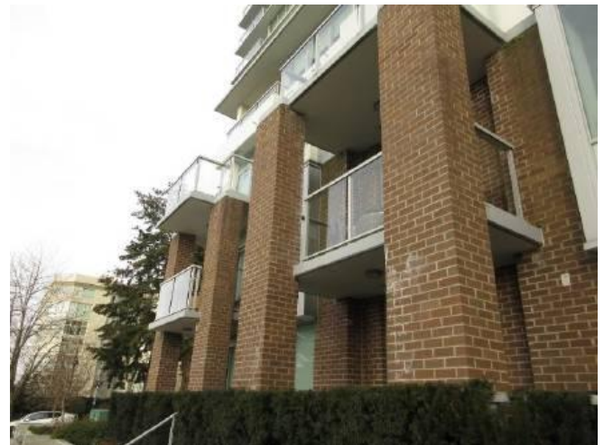
Photo 5: Typical townhouse balconies.
