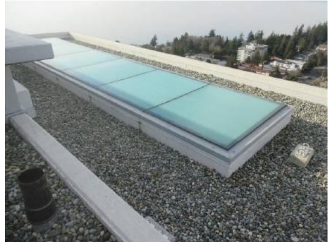
Photo 13: Typical flat roof and skylight.
