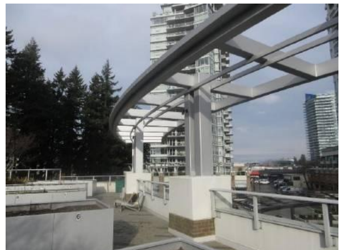
Photo 3: Third floor aluminum trellis.
