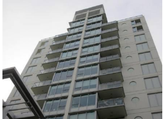
Photo 10: Typical punched and floor to ceiling windows.
