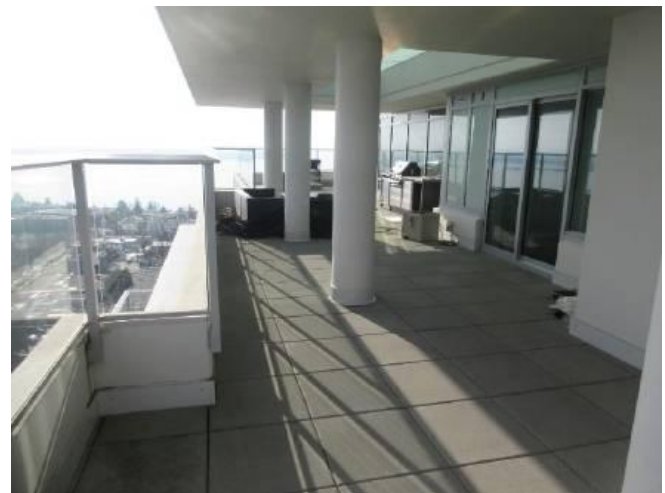
Photo 14: Typical roof deck.
