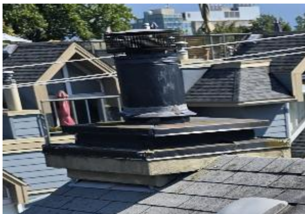
Photo 4.20: Overview of the corroded chimney caps and flue
