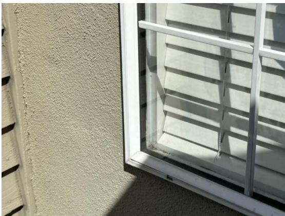
Photo 2.3: Window frame miter not sealed
