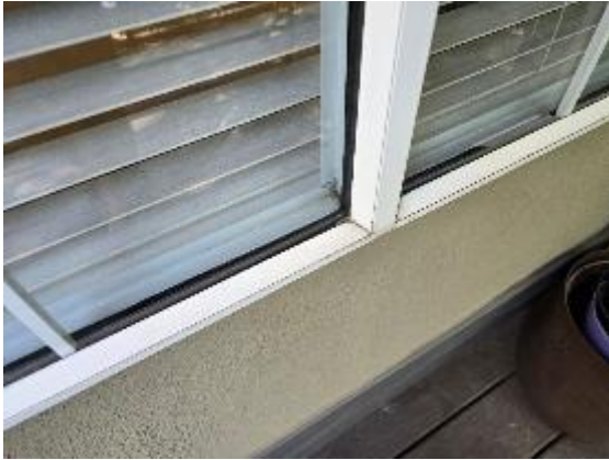
Photo 2.7: Window frame miter not sealed
