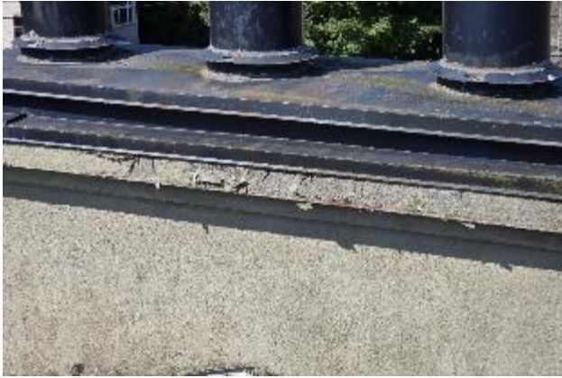
Photo 1.7: Stucco damaged at the chimney level
