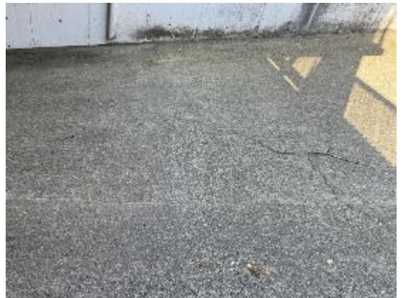
Photo 5.6: Typical cracks on the access ramp
