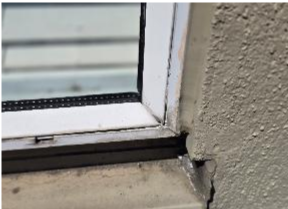
Photo 2.5: Window frame miter not sealed
