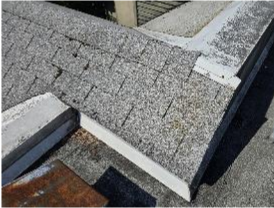
Photo 4.7: Overview of the roof with asphalt shingles
