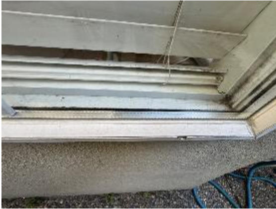
Photo 2.1: Window frame miter not sealed
