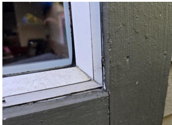
Photo 2.4: Window frame miter not sealed
