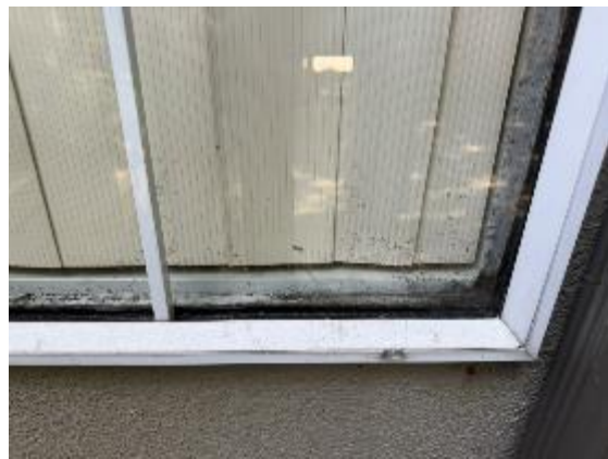
Photo 2.10: Mold at window level
