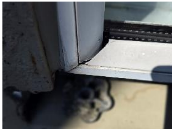
Photo 2.6: Window frame miter not sealed
