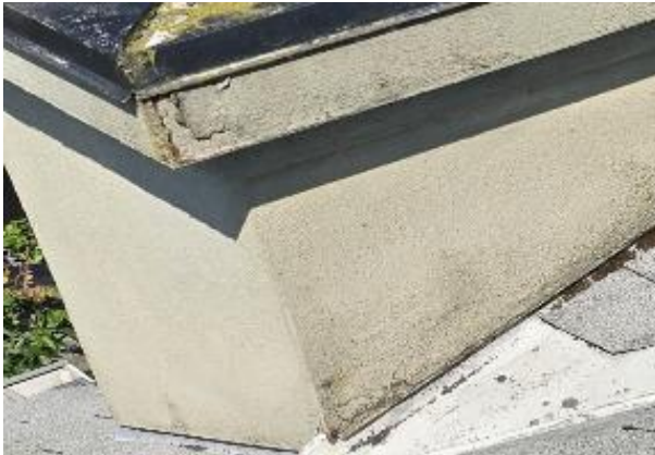
Photo 1.9: Stucco damaged at the chimney level
