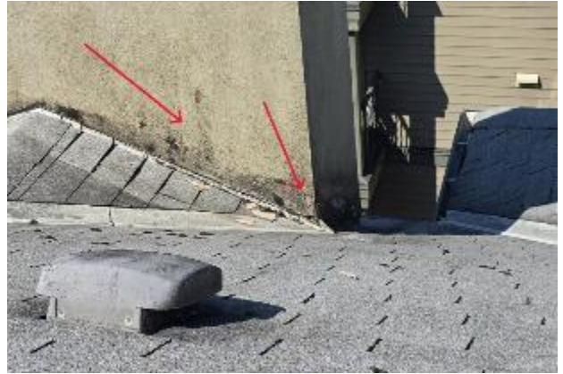
Photo 1.8: Stucco damaged at the chimney level
