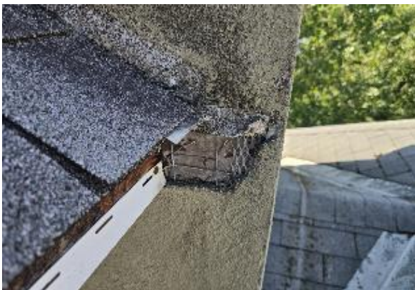
Photo 1.11: Stucco damaged at the chimney level
