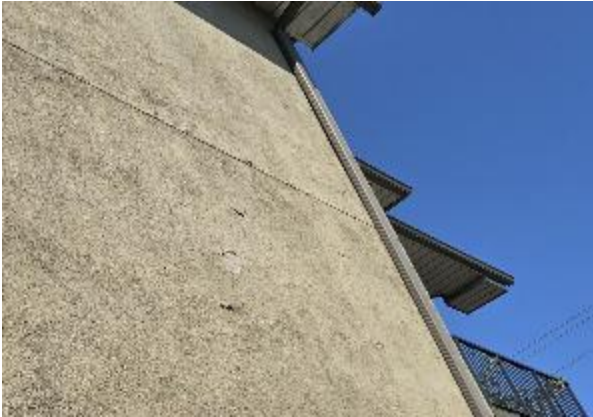
Photo 1.1: Damaged stucco at the wall elevation
