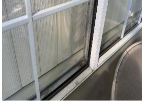
Photo 2.8: Mold at window level
