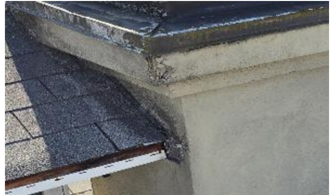
Photo 1.10: Stucco damaged at the chimney level
