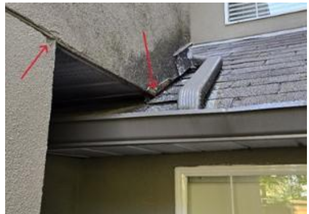
Photo 1.4: Damaged stucco at the end cap and transition strip
