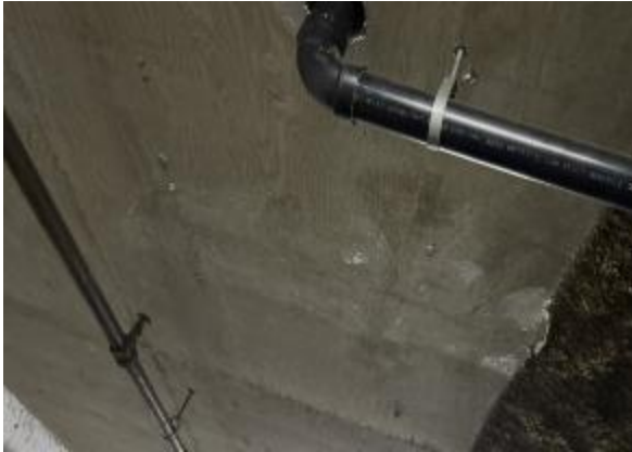
Photo 5.1: Water ingress evidence
