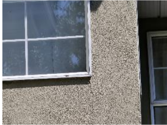
Photo 2.2: Window frame miter not sealed
