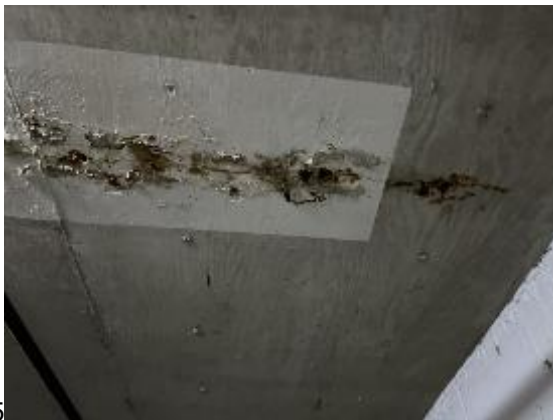
5.5 Photo 5.3: Water ingress staining at parking
