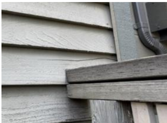
Photo 1.21: Cracked wood siding
