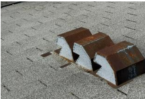
Photo 4.17: Vent caps at the roof elevation
