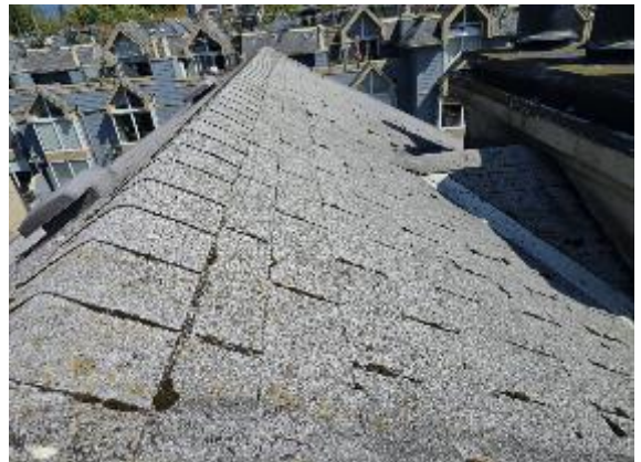
Photo 4.12: Overview of the roof with asphalt shingles
