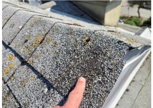
Photo 4.14: View of the roof where the degranulation is visible
