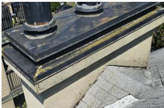
Photo 4.19: Overview of the corroded chimney caps and flue
