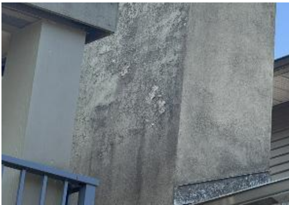
Photo 1.3: Damaged stucco at the wall elevation
