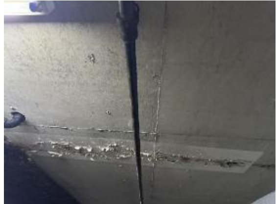
Photo 5.2: Water ingress evidence
