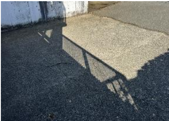
Photo 5.5: Typical cracks on the access ramp
