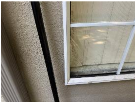
Photo 2.9: Mold at window level
