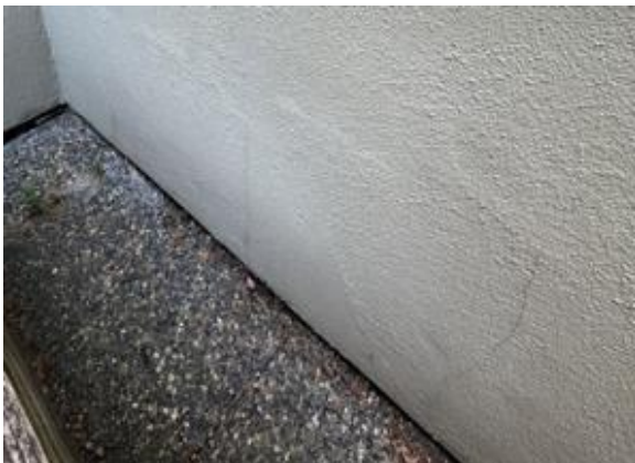
Photo 1.5: Crack stucco at the wall elevation
