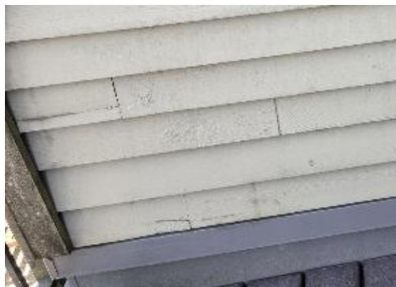
Photo 1.22: Cracked wood siding
