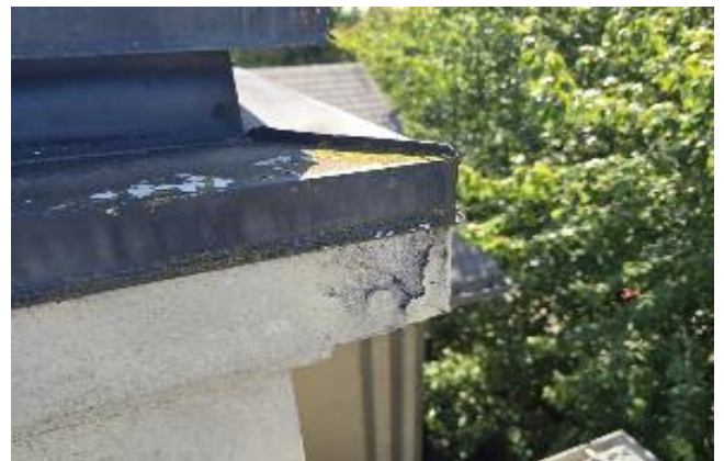
Photo 1.12: Stucco damaged at the chimney level.
