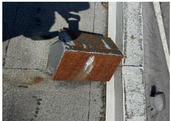
Photo 4.18: Vent caps at the roof elevation
