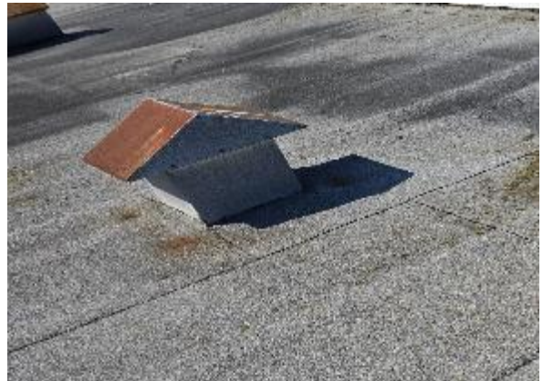
Photo 4.16: Vent caps at the roof elevation
