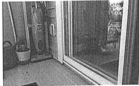
(13) – Proper Upstands at Door Threshold
