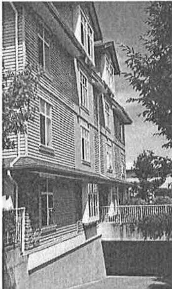
(5) – East View @ Garage Entry Ramp
