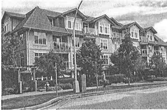
(3) – Front View (South)
