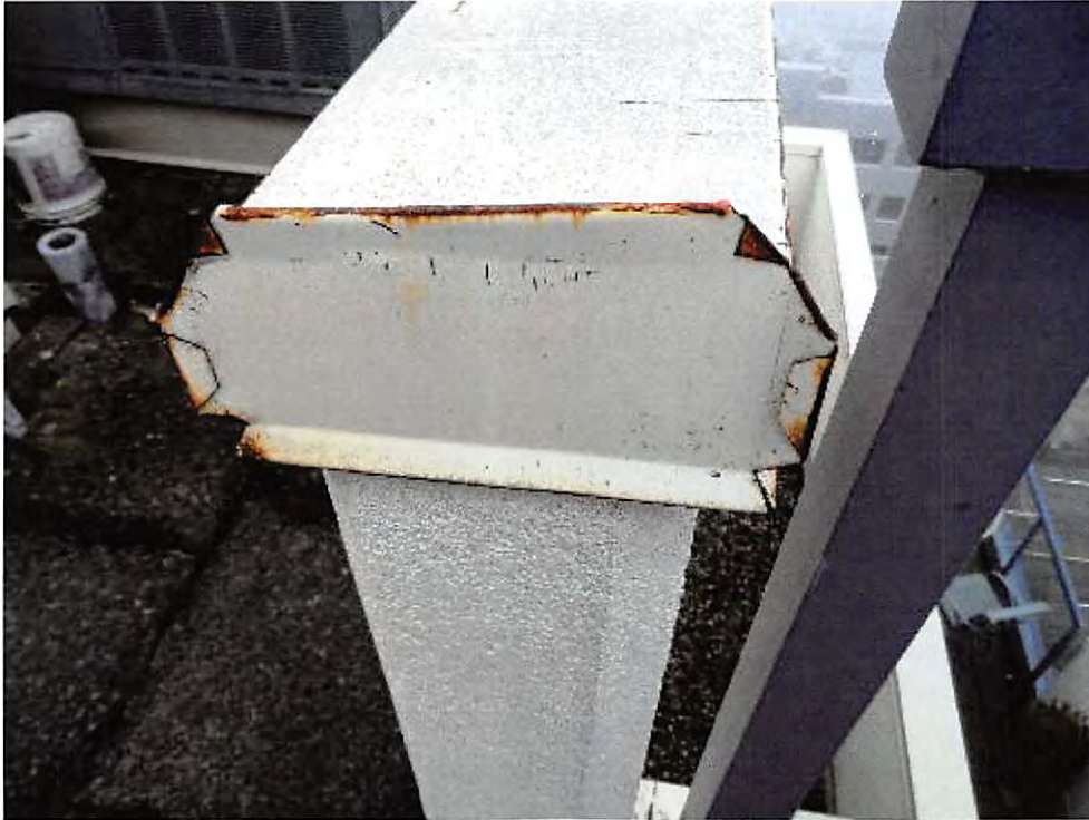
Concrete parapet wall with stucco
