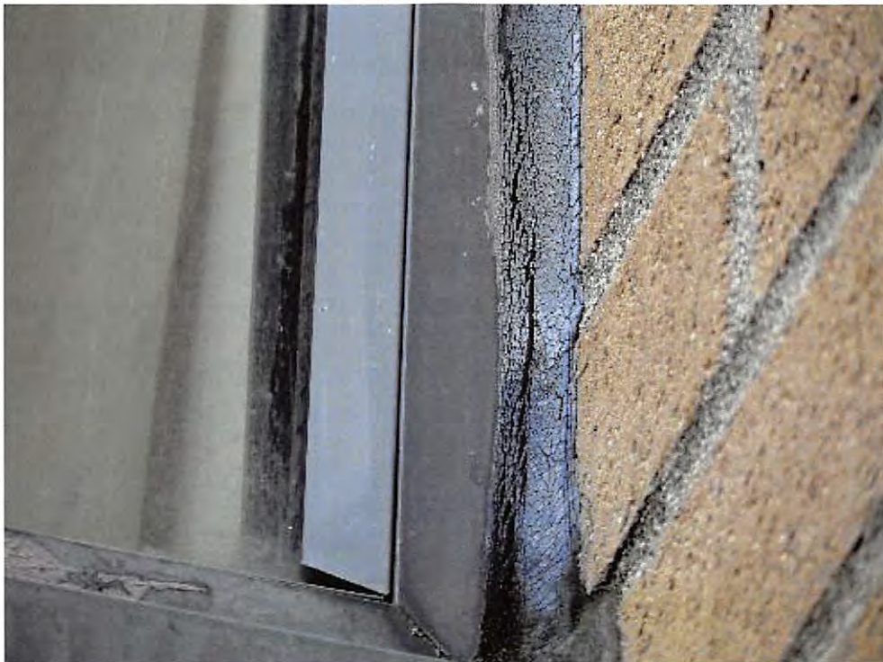
Cracked caulking
