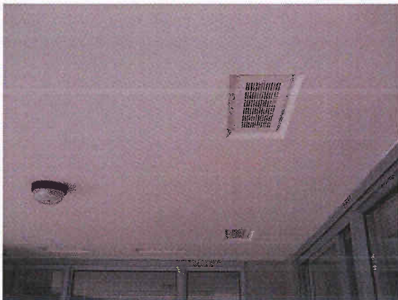
Photo 2.1.9: Typical balcony soffit with louvered exhaust vent grills.
