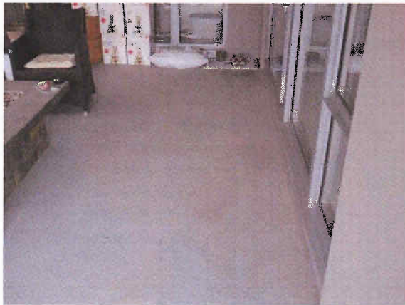
Photo 2.3.1: Typical balcony surface.
