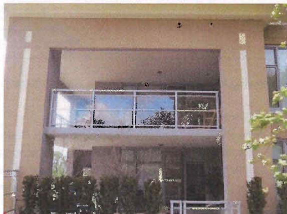
Photo 2.3.4: Typical top mounted balcony guardrail.
