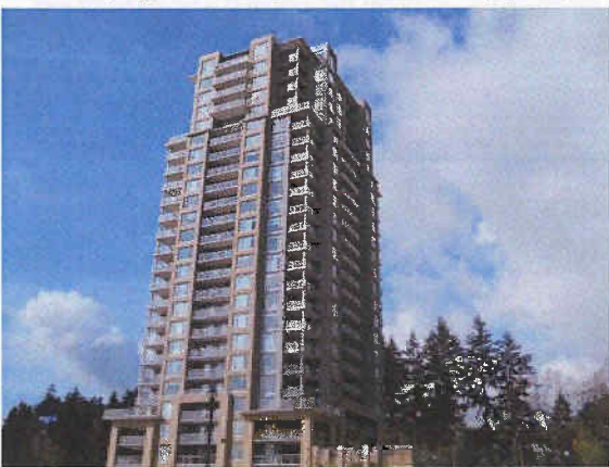
Photo 1.2.1: Partial east and north elevation.
