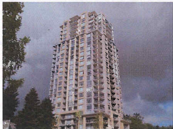
Photo 1.2.2: Partial south and east elevation.
