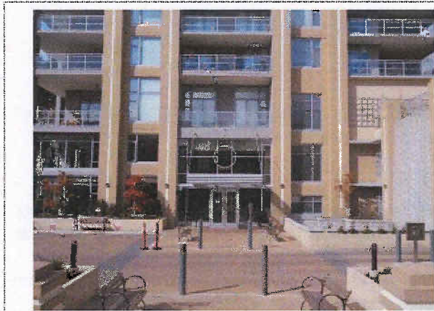
Photo 1.2.3: Front entry at the east elevation.
