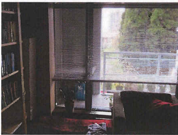
Photo 2.6.1: Interior of the exterior wall at Unit 506.
