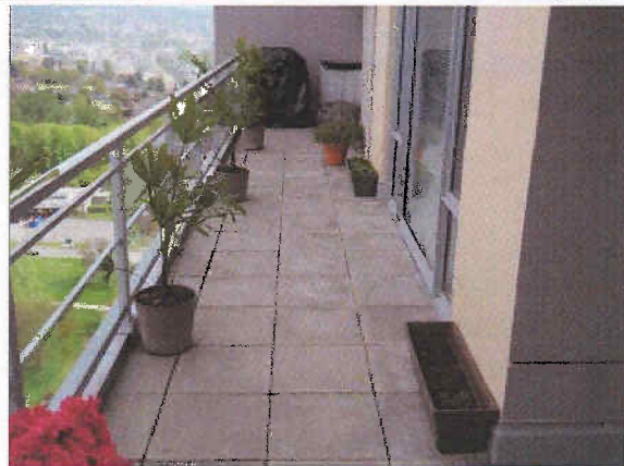
Photo 2.3.2: Typical deck over interior heated living space.
