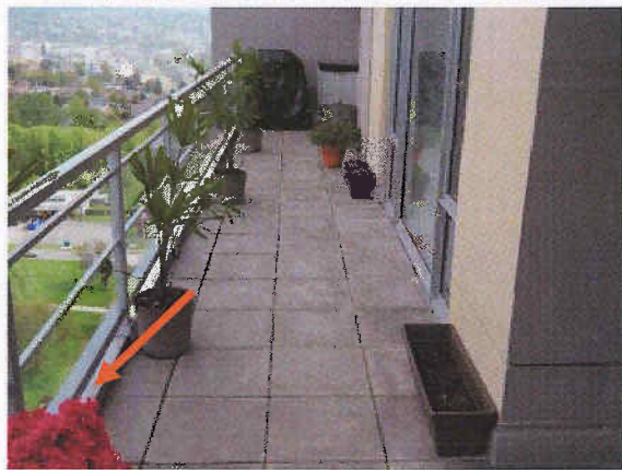
Photo 2.1.8: Typical deck up stand cap flashing.
