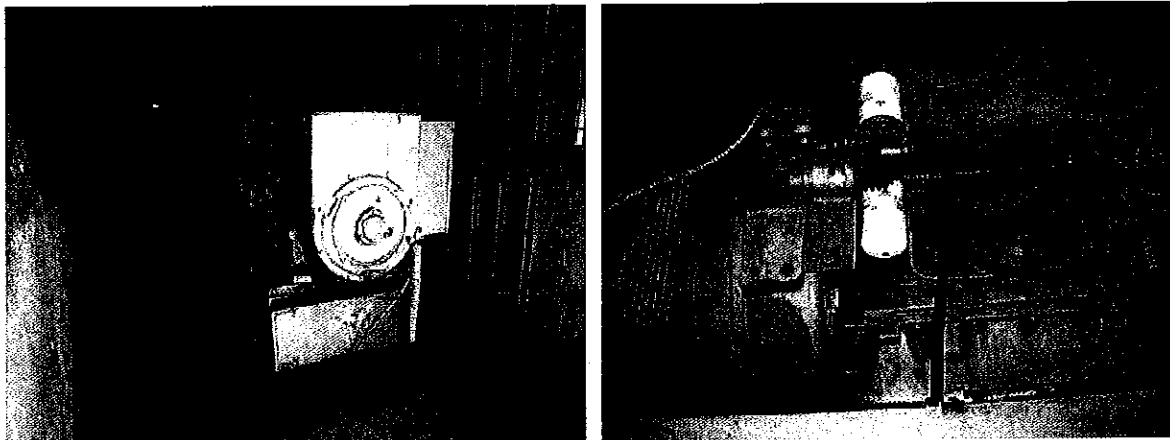
Fig 19. Generator in space above the parkade overhead door (left). Generator side view (right).
