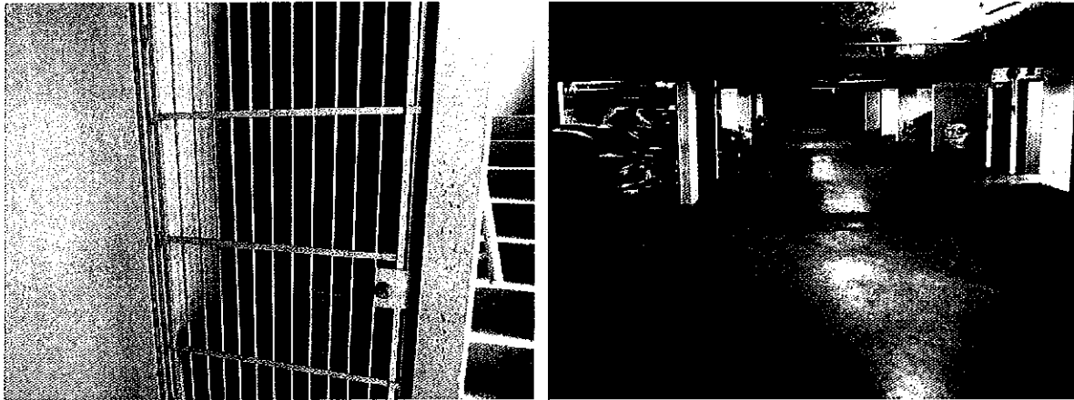
Fig 53. Storage space in a corner of the west stairwell (left). Concrete slab on grade (right).
