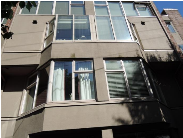
Fig 11 - Upgraded rain screen system and windows (left). Older window and face screened stucco are shown at upper right. Third floor balcony and window upgrades with brick veneer transitions (right).
