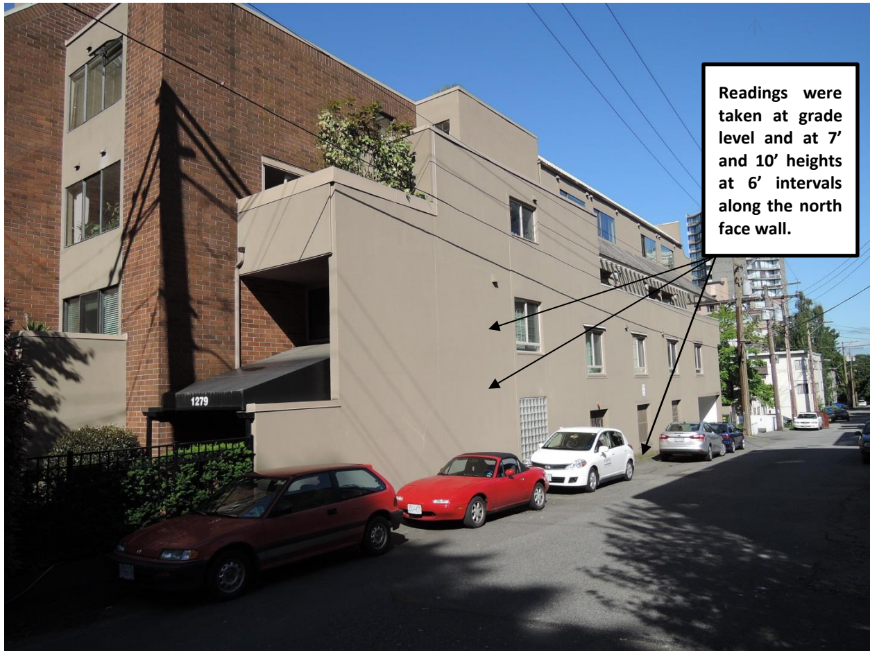
Fig 44 – Readings were taken at various locations on this north wall.
