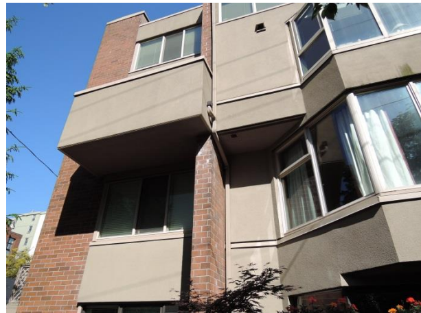
Fig 11 - Upgraded rain screen system and windows (left). Older window and face screened stucco are shown at upper right. Third floor balcony and window upgrades with brick veneer transitions (right).
