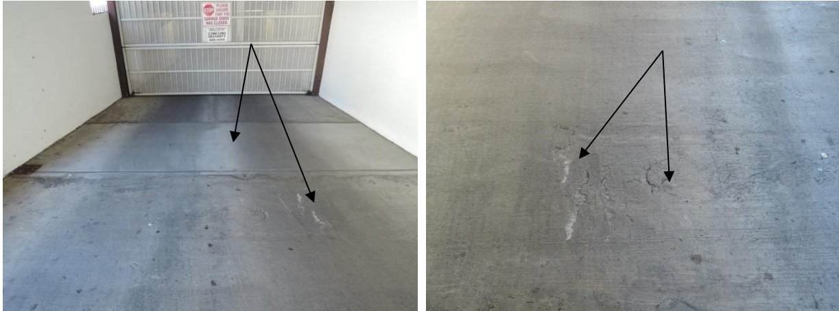
Fig 42 - Replaced ramp section and minor surface deterioration (arrows left). Close up of minor surface deterioration (arrows right).
