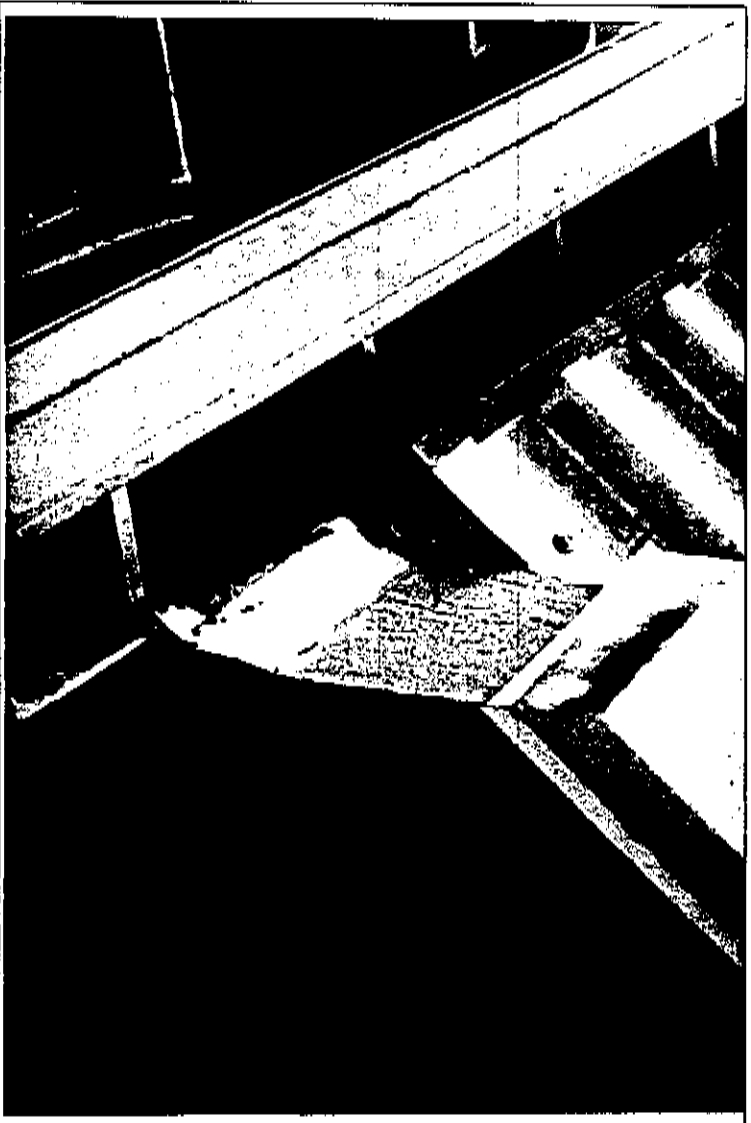
Photo No. 26 – End of a sloped metal roof, revealing a small section of metal flashing installed to direct water into the gutter below. Note the debris in the gutter.
