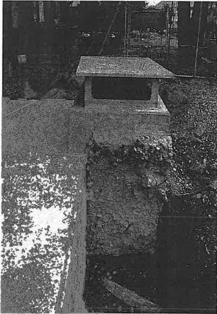
Photo No. 12 and 13- Show the air shaft on the east elevation, which has concrete buildup and cracking. The concrete must be removed, and the cracks injected with epoxy to structurally bond the broken sections.
