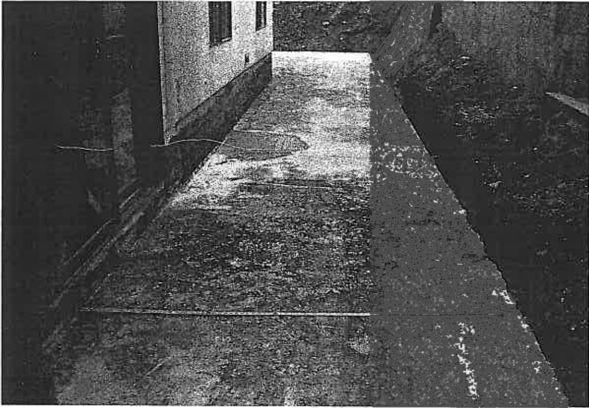
Photo No. 4 - Shows an approximate 32 square foot area where an overlay of the structural repair mortar, Emaco T-430, will be required to fill in the roughness of the suspended slab. This photograph was taken looking south from the west elevation, next to the mid-elevation patio.
