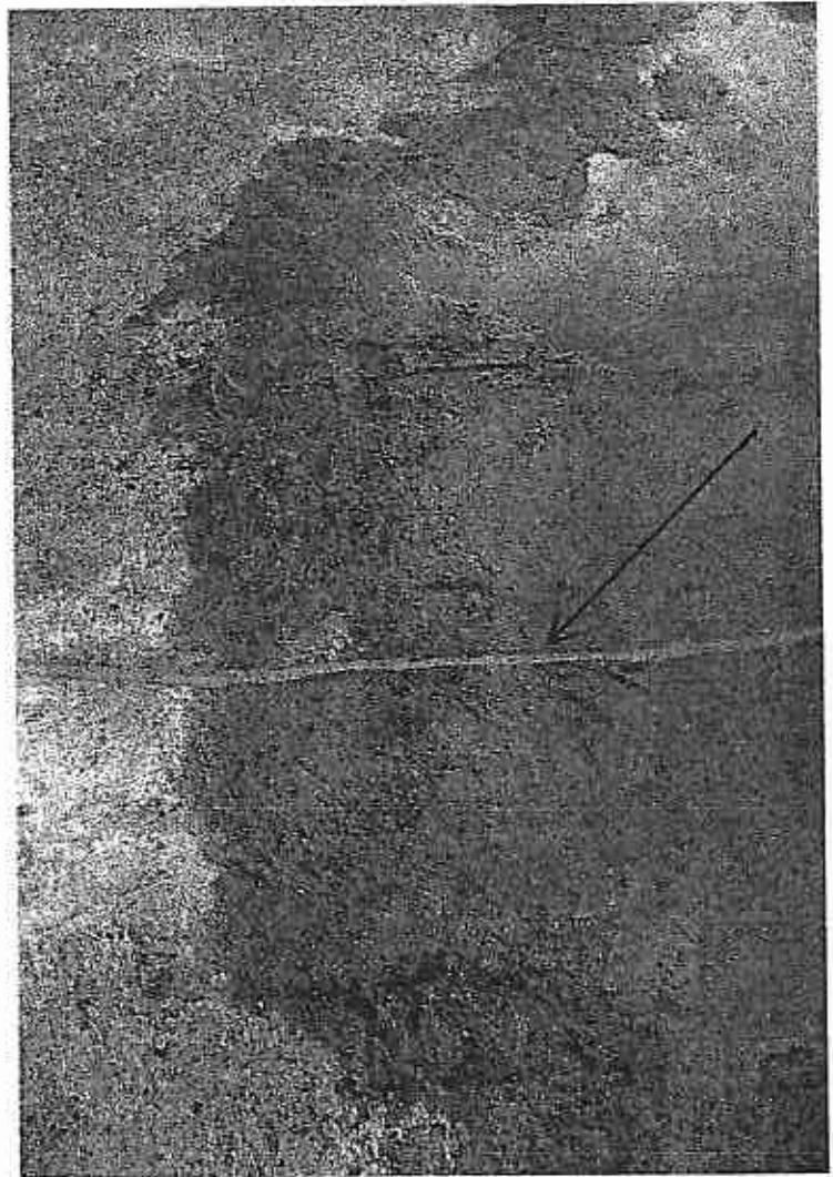
Photo No. 14 and 15 - Show caulking of cracks after V-grooving. The caulk sealant used is Sonneborn NP-1.
