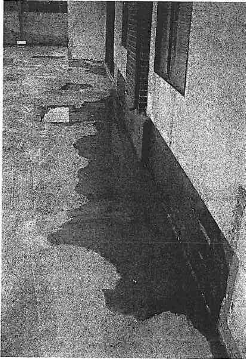
Photo No. 16 - Shows ponding of water against the building. This area should be resloped with the specified mortar.
