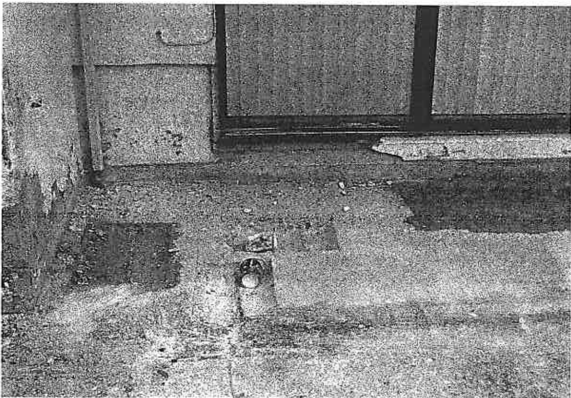
Photo No. 2 and 3 - Show areas of delaminated concrete on the west side of the main entrance suspended slab where the Emaco T-430 structural repair mortar will be utilized for the infill.
