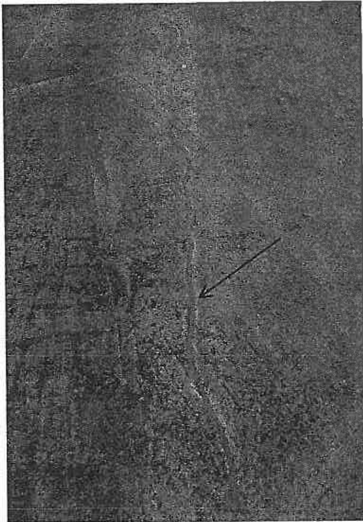
Photo No. 14 and 15 - Show caulking of cracks after V-grooving. The caulk sealant used is Sonneborn NP-1.
