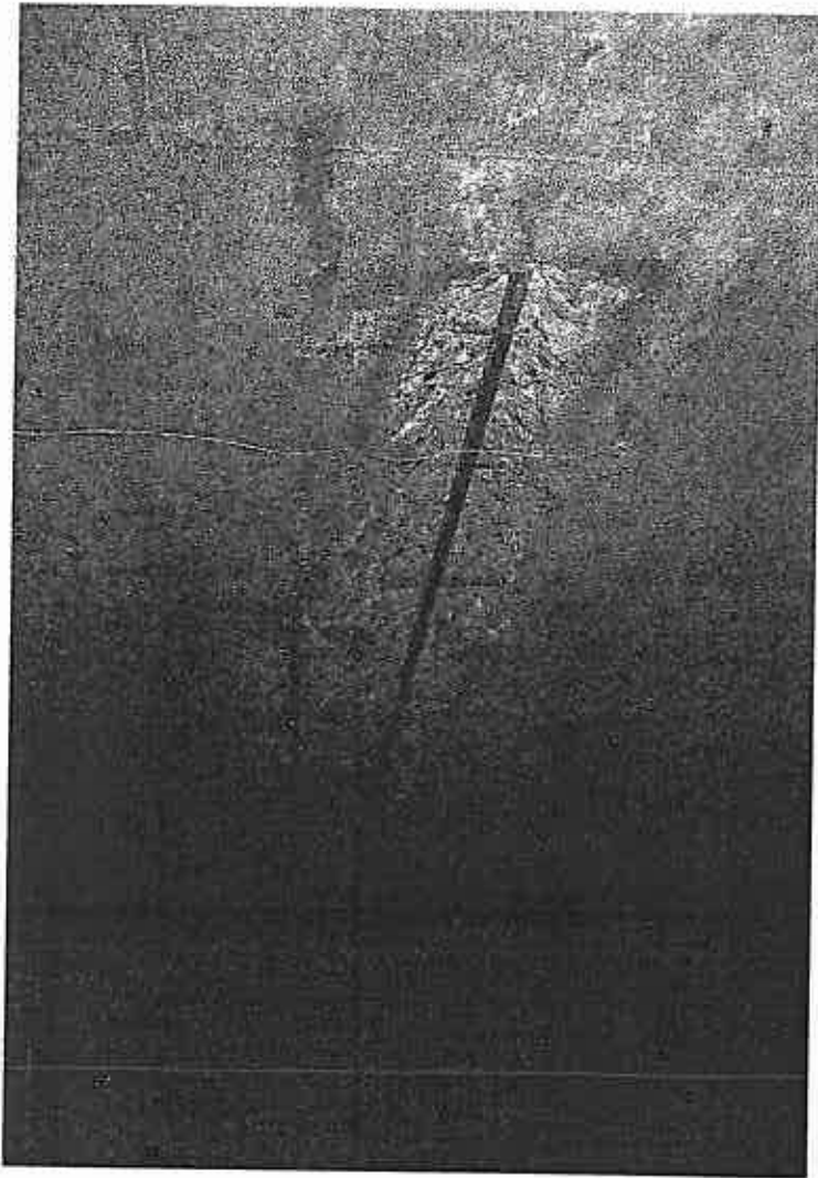
Photos No. 7 & 8 – Show typical areas being chipped of the existing delaminated concrete and preparation for repair.
