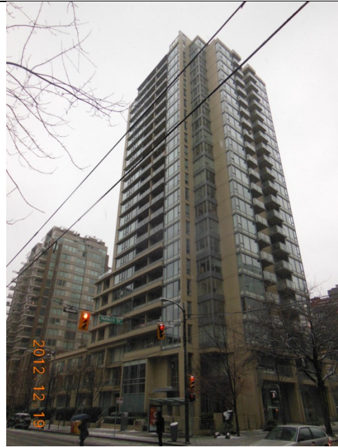
Photograph 3.2 - East and North Elevations
