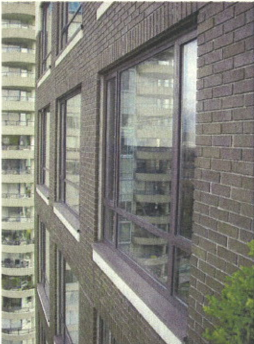
Photo 07 Typical punched window assembly in pre-fabricated panel
