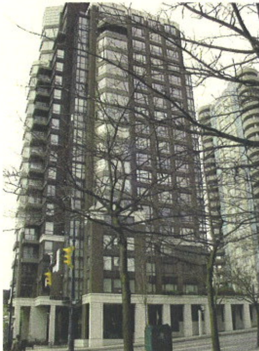
Photo 03 Southeast Elevation - Burrad Street
