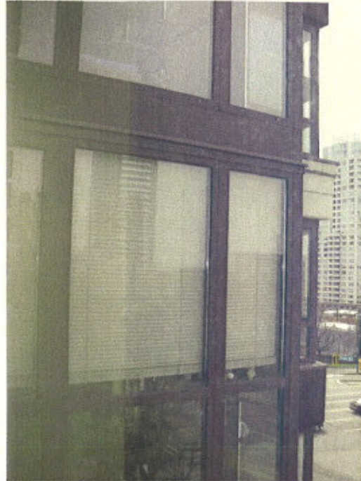
Photo 22 Typical window wall assembly at enclosed balcony
