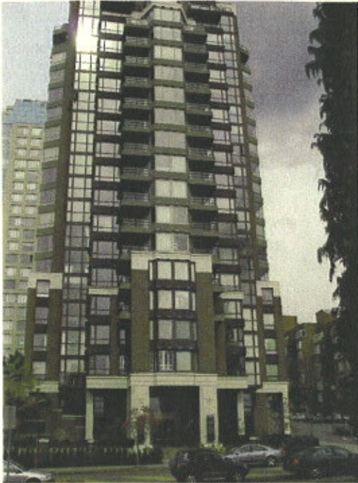
Photo 01 Southwest Elevation - Pacific Street
