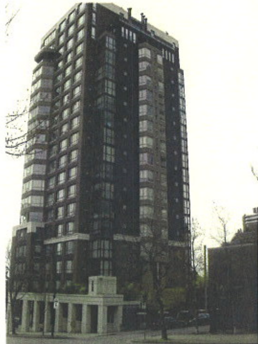
Photo 04 Northeast Elevation - Lane
