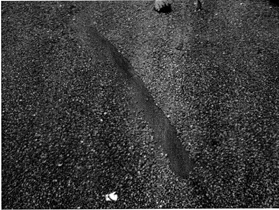
old repair OK
