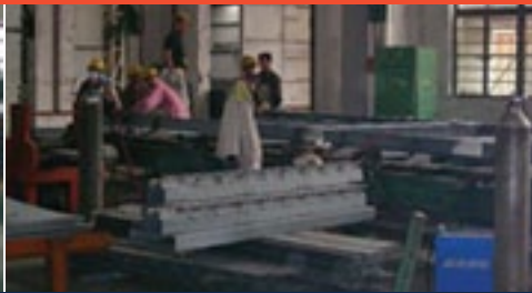
Fabricating the base frame
