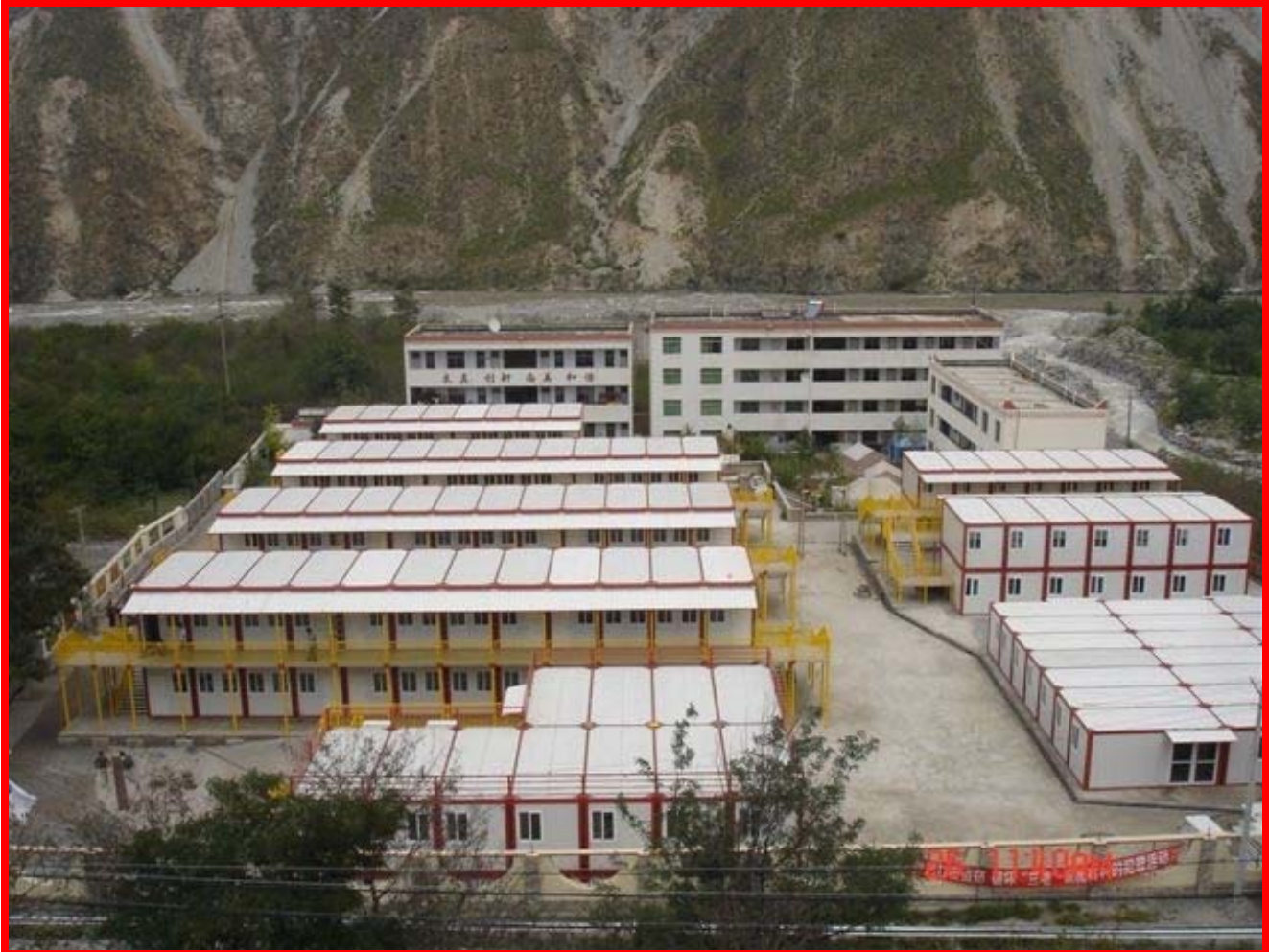
Disaster Relief China; modules were later dismantled and used as schools in the region
