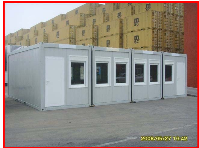
Four units assembled to make a 20' x 32' room
