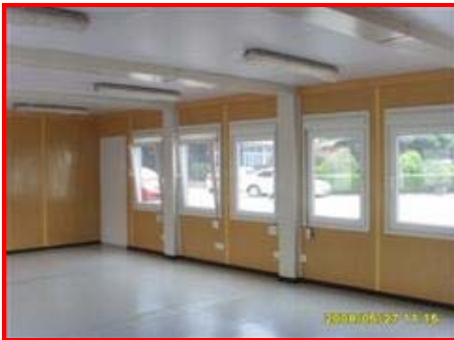
Four units assembled to make a 20' x 32' room
